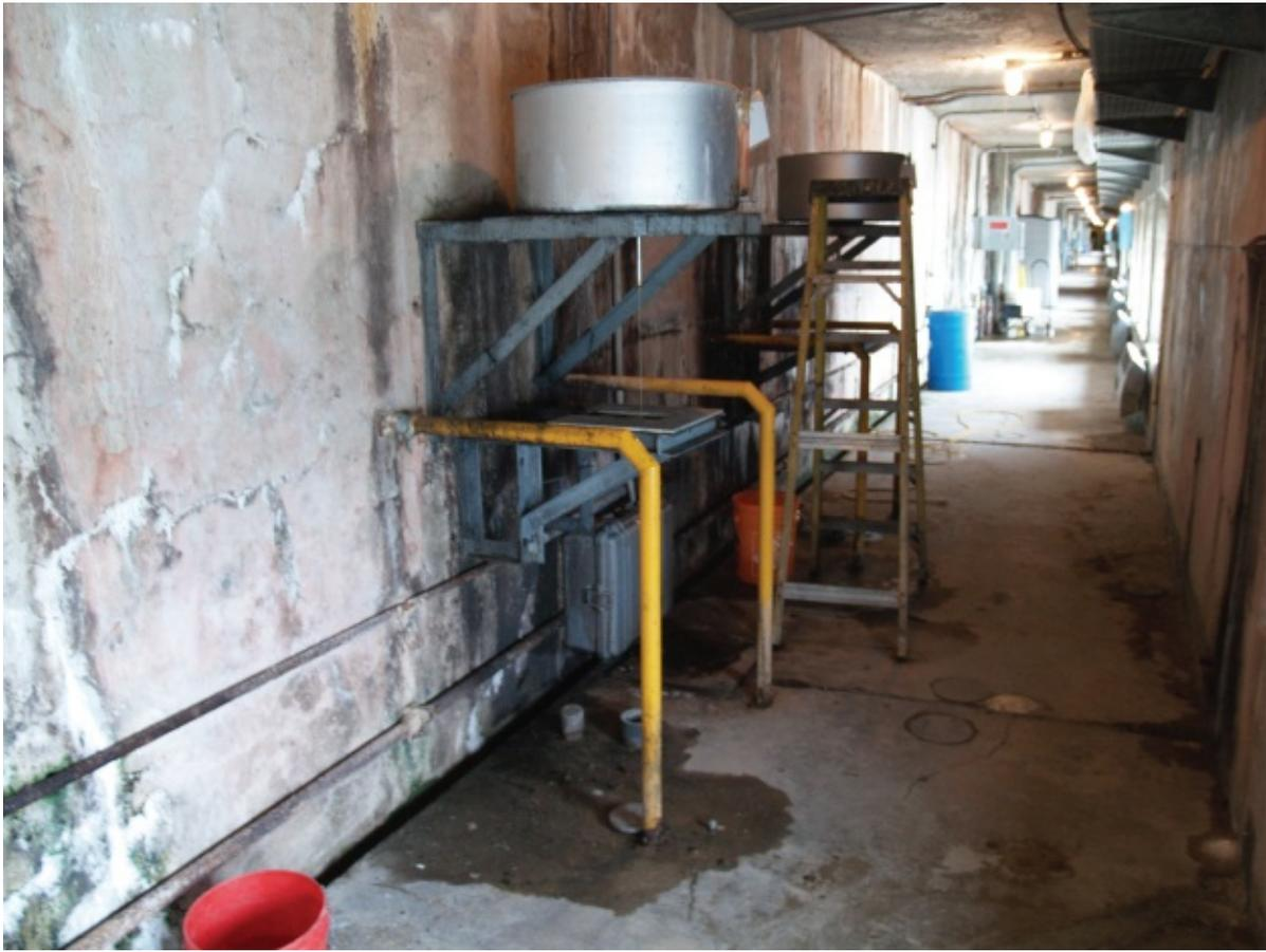
**Figure 11.18** Inverted plumbline installations in one of the galleries of the Intake structure of a generating station (with brackets bolted to concrete wall).
