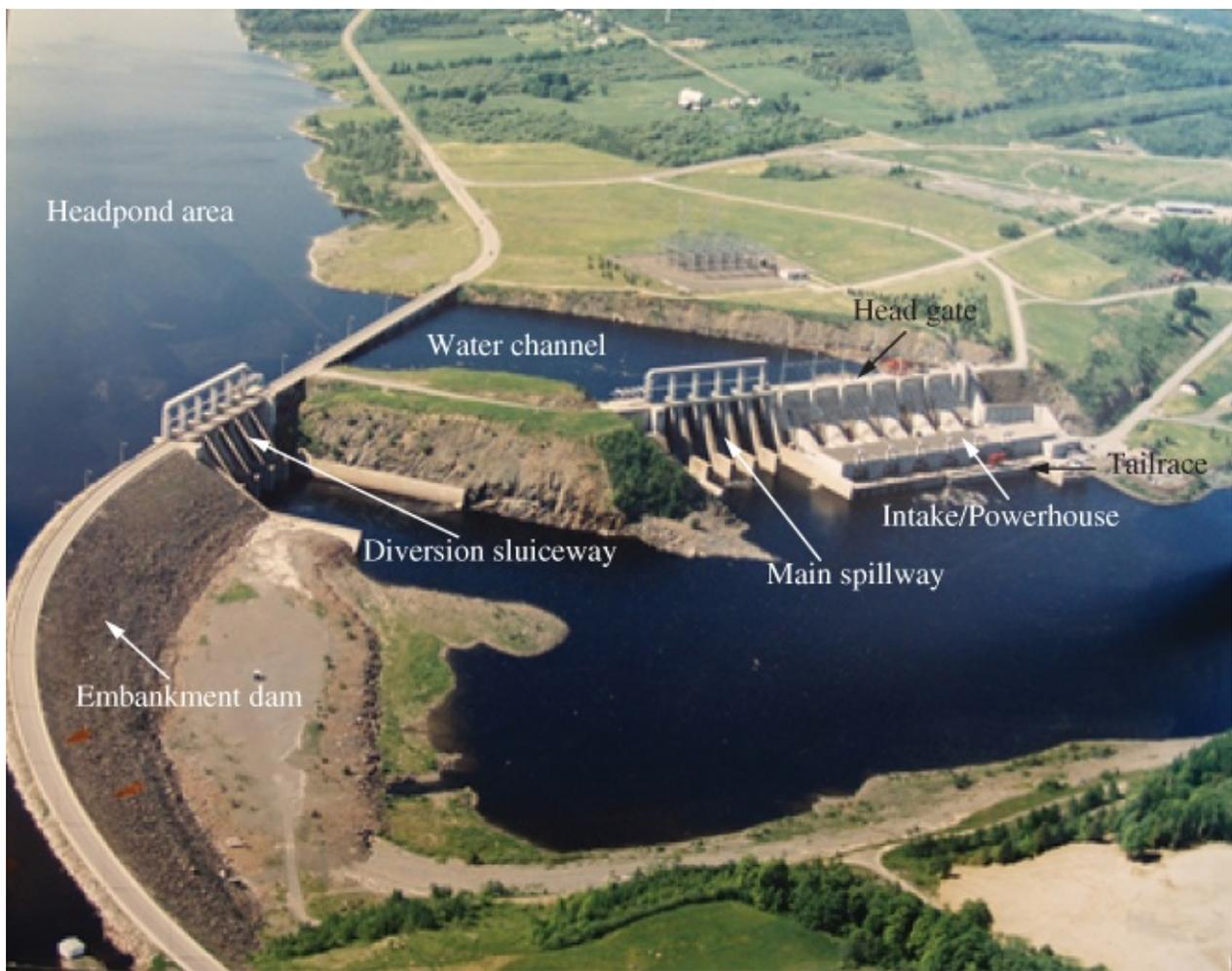
**Figure 9.8** Main features of a typical hydroelectric generating station. *Source:* Background image is reproduced by permission of NB Power.
