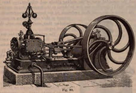
annexed Fig. 80, adapts itself to small steam-motors. It consists of a rectangular slide-bar upon the four longitudinal surfaces of which, the motion-block slides. This motion bar is supported in a very ungainly manner.
