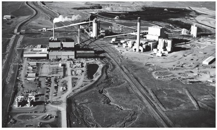
Fig. 27 This energy complex in the northern U.S. includes four coal-fired steam systems, ranging from 80 to 330 MW, installed over a 25-year period.
