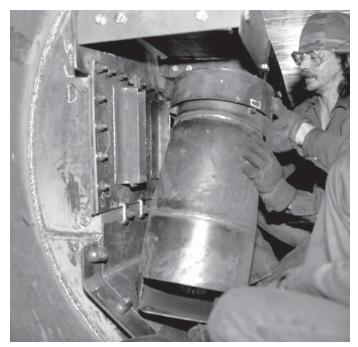
Fig. 23 Cyclone steam separator installation.
