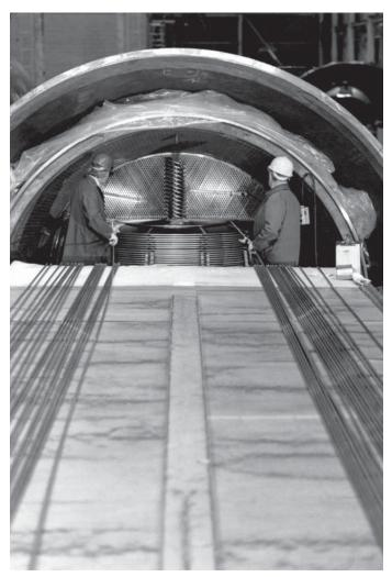
Fig. 18 Installation of tubing.
