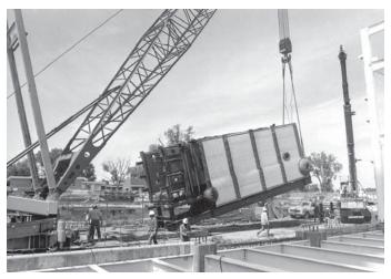
Fig. 10 Field assembly of a Towerpak<sup>®</sup> boiler.
