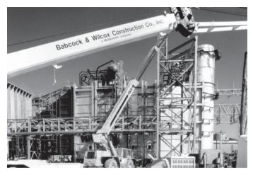
Fig. 6 Rapid installation of modular components minimizes schedules.
