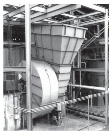
Fig. 17 Forced draft centrifugal fan for a 364 MW outdoor unit.
