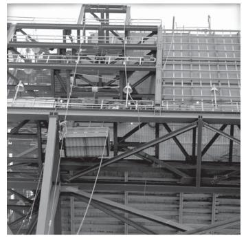
Fig. 8 Installation of catalyst blocks.
