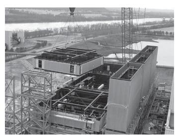
Fig. 2 SCR retrofit construction.
