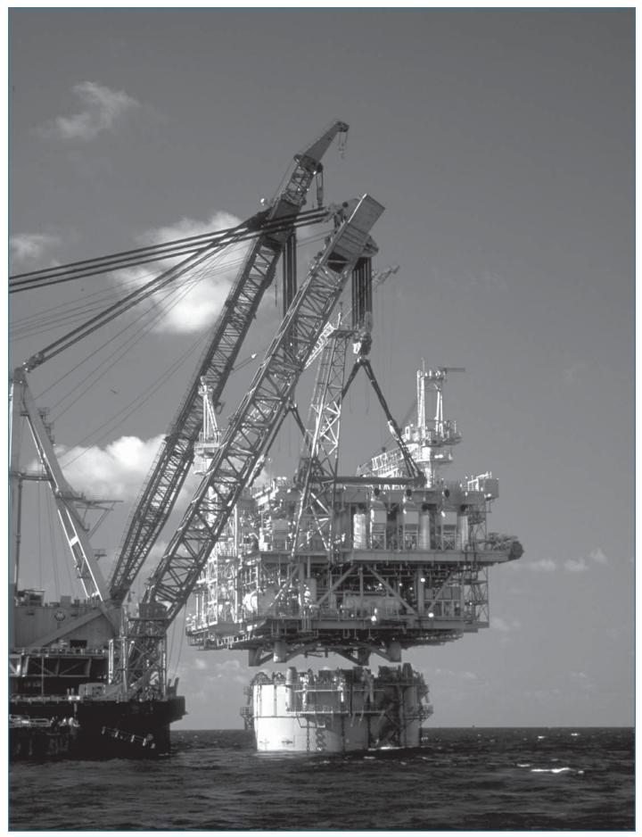
Fig. 1 Deepwater oil and gas fields require new floating technology facilities like this Spar being installed in the Gulf of Mexico.
