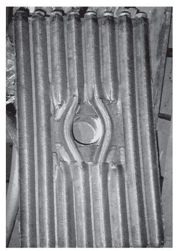
Fig. 13 Laser clad sootblower opening.
