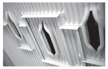
Fig. 17 Burner and secondary air port windbox attachments.
