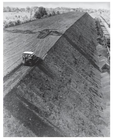
Fig. 16 Long-term coal storage – typical example of thorough packing with minimal size segregation. This pile contains about 200,000 t of coal.
