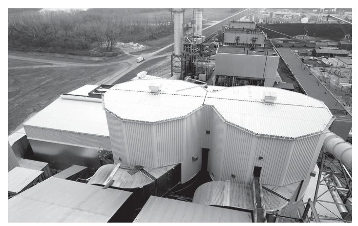
Fig. 12 B&W's SDAs and fabric filter baghouse provide an integrated SO<sub>2</sub> and particulate removal process.
