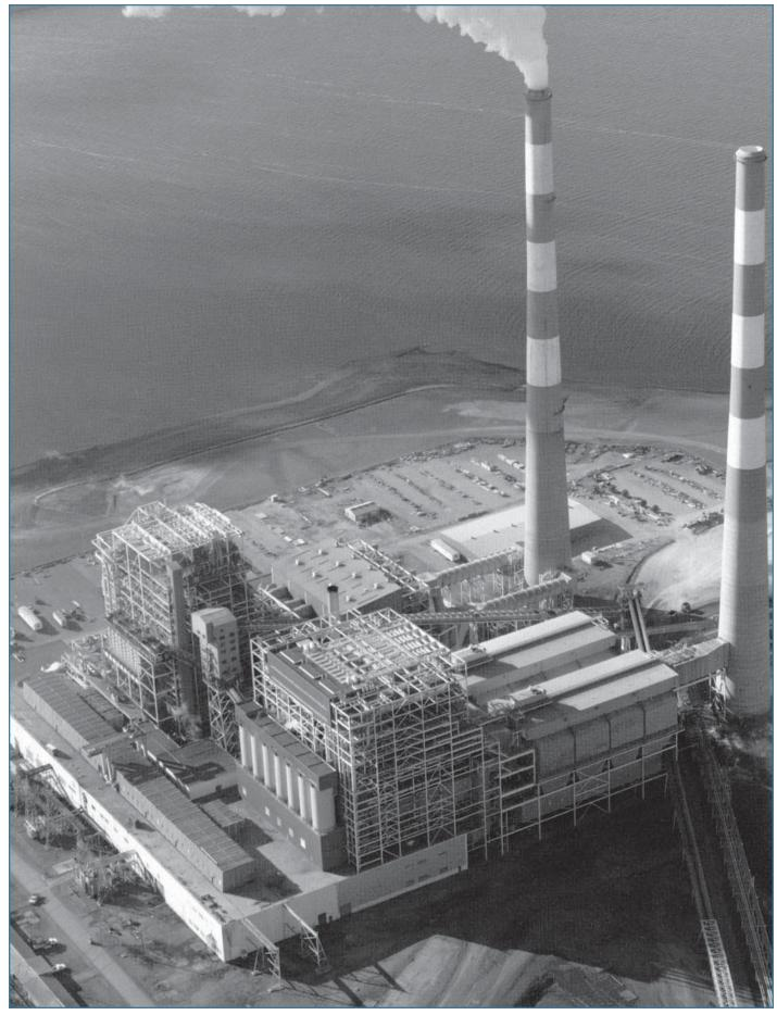
Two coal-fired boilers: one 685 MW pulverized coal unit and one 844 MW unit with Cyclone™ furnaces.
