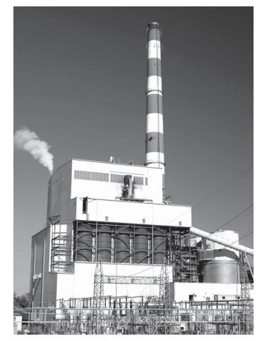
Fig. 27 B&W boiler with SO<sub>2</sub>, NO<sub>x</sub>, and particulate control systems.
