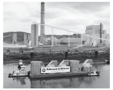
Fig. 5 Large scrubber modular components on a barge.
