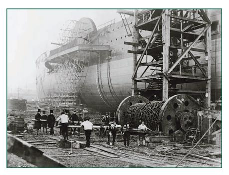
The *Great Eastern*, the first attempt at a large luxury steamship, used two 56-foot side-wheels and 10 boilers to propel its 680-foot-long iron hull with the power of steam. It took 2,000 workers four years, from 1854 to 1858, to construct the luxurious steamship on England's River Thames.
