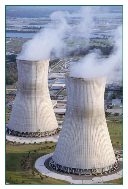
It is steam, not smoke, that drifts from the cooling towers of nuclear power plants. The energy produced by nuclear fission makes the steam that drives the turbines to generate electricity. between the steam power of today and that of the last century is that today steam power is carefully monitored by computers, eliminating errors in steam pressure and water levels.
