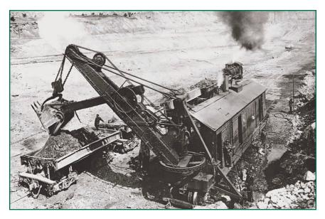
The mining industry profited immensely from the invention of the steam engine. Originally harnessed to pump standing water from underground mines, steam was also utilized to power the shovels used in strip mining. The advancements of steam engines in mining meant that even children could do the work, creating issues about child labor laws.
