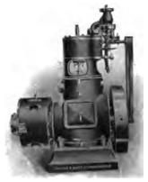
FIG. 143.—SINGLE CYLINDER ENGINE AND OVERHUNG DYNAMO, BY NESSRS. MATHER AND PLATT, LIMITED.
