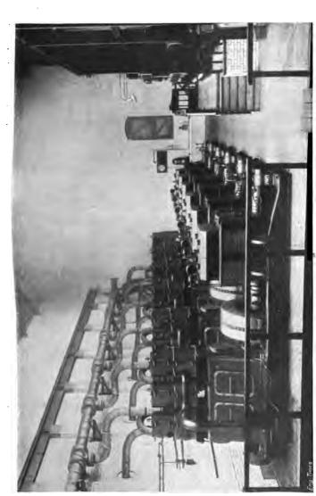
FIG. 9.--VIEW SHOWING SIX SETS OF THREE-CRANK TANDEM COMPOUND "BELLISS" ENGINES AND DYNAMOG INSTALLED AT THE WATERLOO AND CITY ELECTRIC RAILWAY GENERATING STATION.
