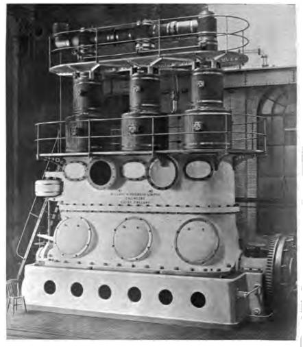
FIG. 116.-WILLANS' CENTRAL-VALVE TRIPLE-EXPANSION ENGINE, CAPABLE OF DEVELOPING 3,000 H.P.
