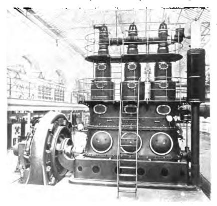
FIG. 136 .---- 1,075 B.H.P. "WILLANS" HIGH SPEED ENGINE DIRECT CONNECTED TO DYNAMO.
