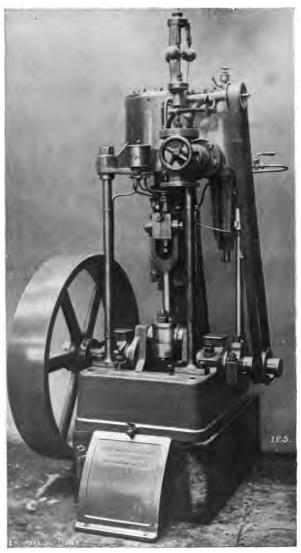
FIG. 30.—ERNEST SCOTT AND MOUNTAIN'S SINGLE CYLINDER HIGH SPEED ENGINE. "OPEN" TYPE.
