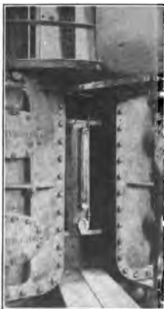
FIG. 19.—Typical condenser barometer for steam turbine operation.
