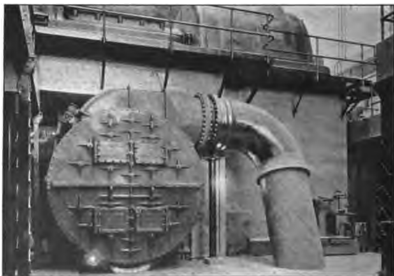
FIG. 237.—The condenser and a portion of the 42 inch discharge salt water pipe for the new 15,000 kw. turbo generator, station A, San Francisco, Pacific Gas and Electric Company.
