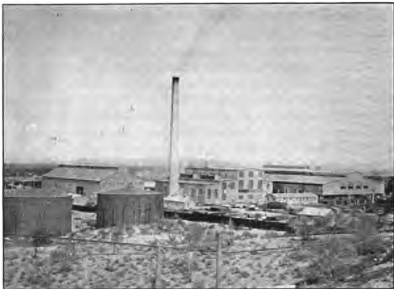
FIG. 214.—Exterior view of power plant of New Cornelia Copper Co., Ajo, Arizona, showing tapered construction of reinforced concrete stack 220 feet high.
