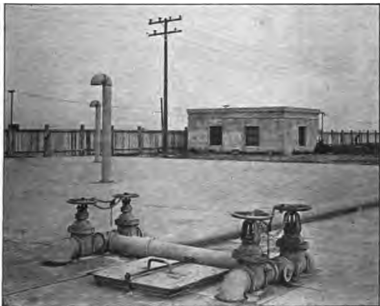
FIG. 42.—A close up view of the filling pipes for the oil storage reservoirs of the Southern California Edison Company's Long Beach Plant. These valves are under control of the oil company from whom the oil is purchased.
