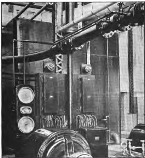
FIG. 202.—Venturi meter for measuring water supply at the Long Beach Plant of the Southern California Edison Company shown installed on piping in upper right center.
