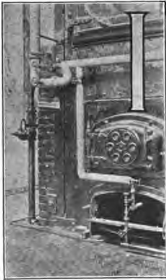
FIG. 178.—Boiler front—oil fired; showing gage for measuring chimney draft.
