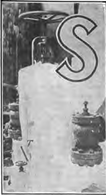
FIG. 50.—Thermometer inserted for superheat measurement.
