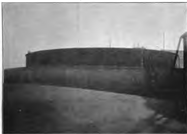
FIG. 124.—Main oil storage tanks at Station C, Pacific Gas and Electric Company, Oakland, California. Tank in foreground is set low for fire protection purposes, while tank in rear is surrounded by concrete retaining walls.
