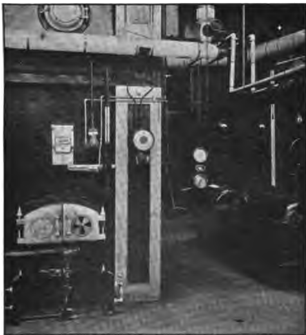
FIG. 185.—Steam flow meter and draft gage on the left with Venturi meter on the right. This apparatus is at the Redondo Steam Plant of the Southern California Edison Company.
