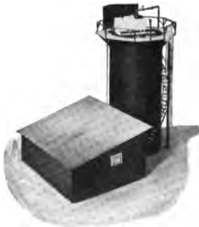
FIG. 4.—Measuring and purifying tank for water supply at Redondo plant.
