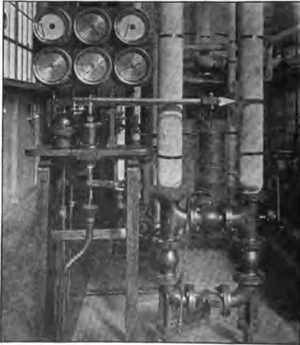
FIG. 140.—On the left may be observed oil-to-burner Moore regulator controlling the steam pressure and the oil pressure while on the right may be seen the damper controller that works by hydraulic cylinder actuation at the Arizona Power Company, Phoenix, Arizona.
