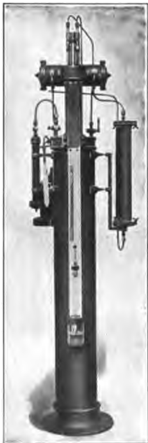
FIG. 169.—A carbon dioxide recorder.
