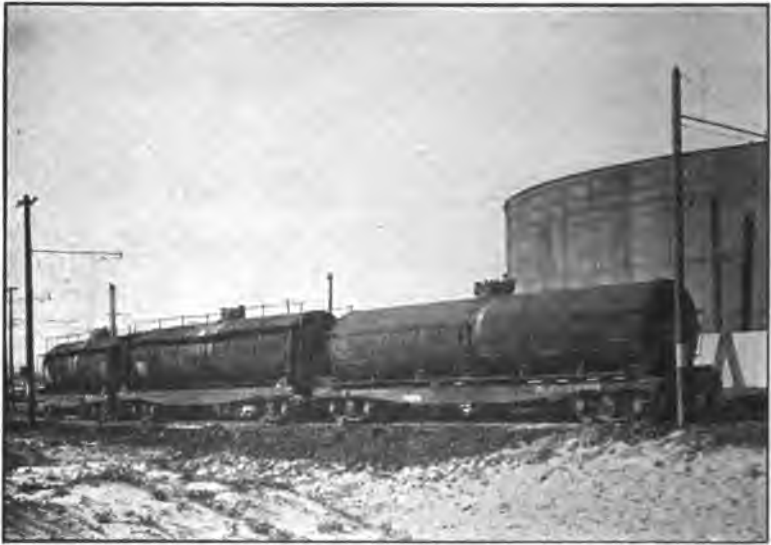
FIG. 123.—The cars are shown on the unloading track of the Redondo Steam Plant of the Southern California Edison Company and the oil is emptied from them into the flume which runs beside the tank; thence it goes into a small underground tank from which it is pumped into the main storage tank.
