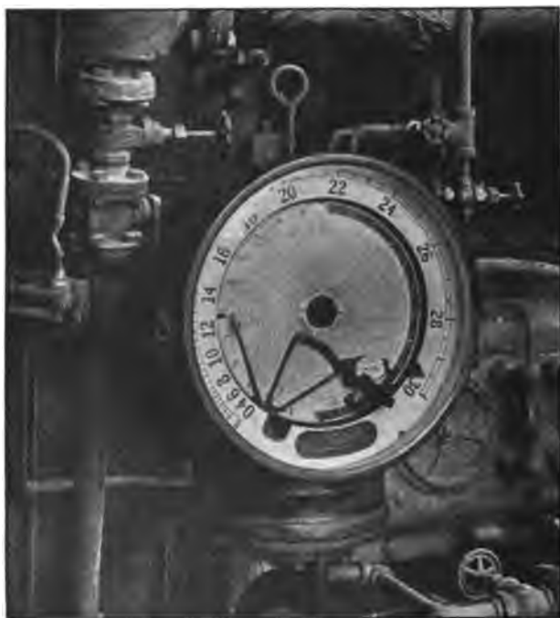
FIG. 186.—Steam flow meter with integrating device for registering total quantity of steam passed.
