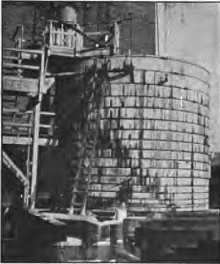
FIG. 75.—Water softening plant at the Sierra and San Francisco Power Company's 27,000 kw. oil burning station. The use of pure water free from scale forming matter is the first requisite toward keeping boilers clean.
