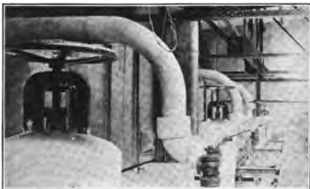
FIG. 32.—Superheated steam approximately obeys simple thermodynamic laws. (Superheated steam ducts of station C of the Pacific Gas & Electric Company in Oakland.)
