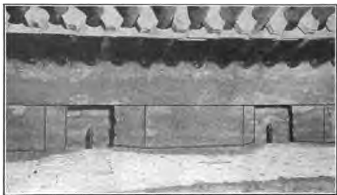
FIG. 205.—Checkerwork and housings installed around burners.
