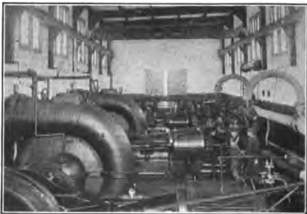
FIG. 33.—Saturated steam obeys not at all the simple laws of thermodynamics. (Circulating water pumps operated by saturated steam at the Redondo plant of the Southern California Edison Company.)
