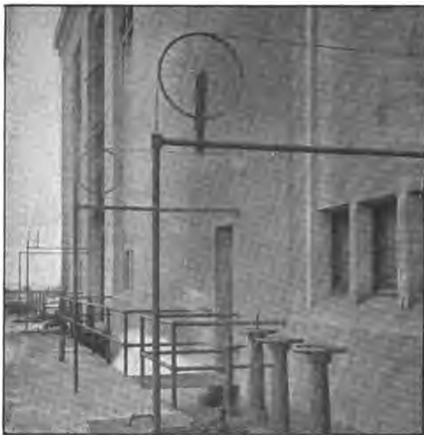
FIG. 177.—View of the float arrangements, showing the valves which control the inlet and outlet of oil from storage tanks of Long Beach Plant, Southern California Edison Company.
