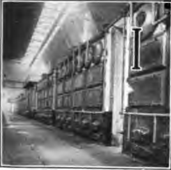
FIG. 68.—A battery of fifteen boilers oil-fired, requiring but two men for their operation.
