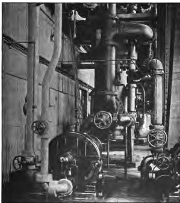
FIG. 240.—Auxiliary apparatus, including centrifugal feed pump and feed water heater at Station C., Pacific Gas and Electric Company, Oakland.
