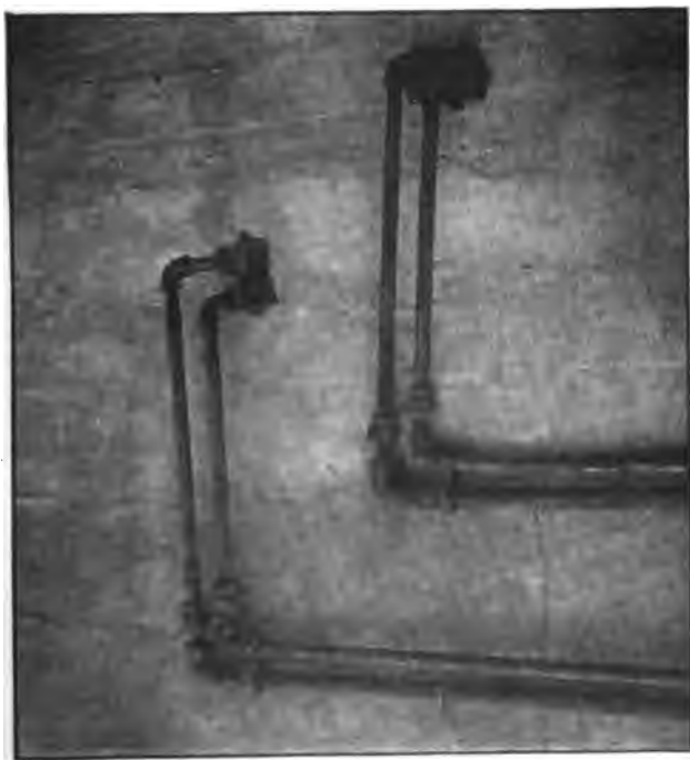
FIG. 96.—Typical burners and control pipes ready for installation.
