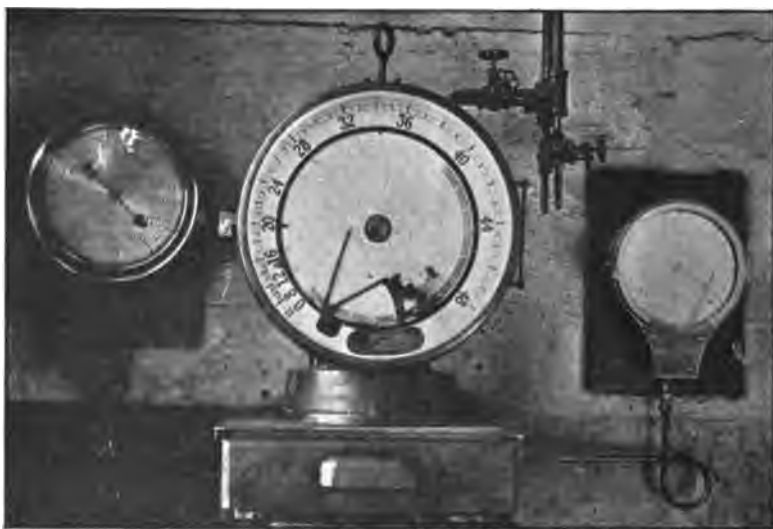
FIG. 43.—Steam flow meter, recording pressure gage and indicating pressure gage, Station C, Pacific Gas and Electric Company, Oakland, California.
