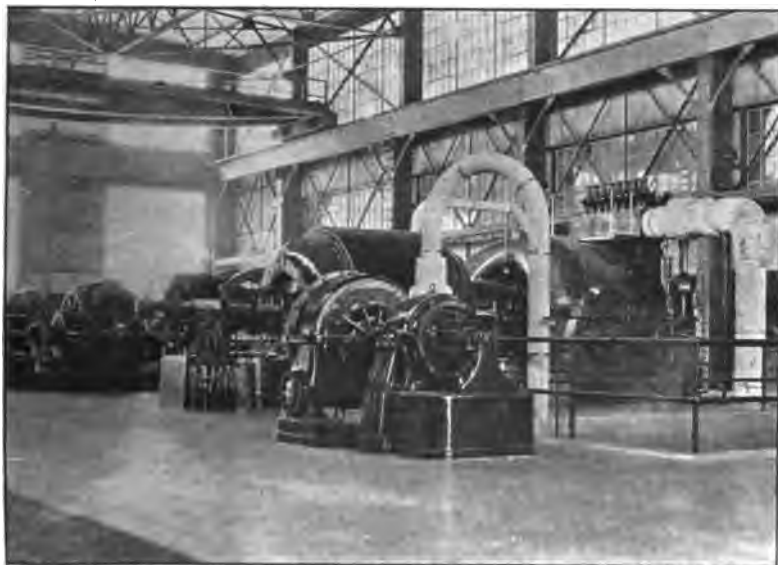
FIG. 216.—Turbine room, New Cornelia Copper Co., Ajo, Ariz., showing an auxiliary exciter unit in the foreground, one of the turbo-generators, and four motor generator sets in the background. Three of these sets are in continuous operation, and carry a total load of 30,000 amperes at 160 to 170 volts on the d.c. side, 24 hours a day.
