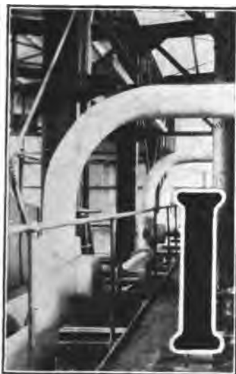
FIG. 48.—Piping in boiler setting where superheat temperatures are taken.
