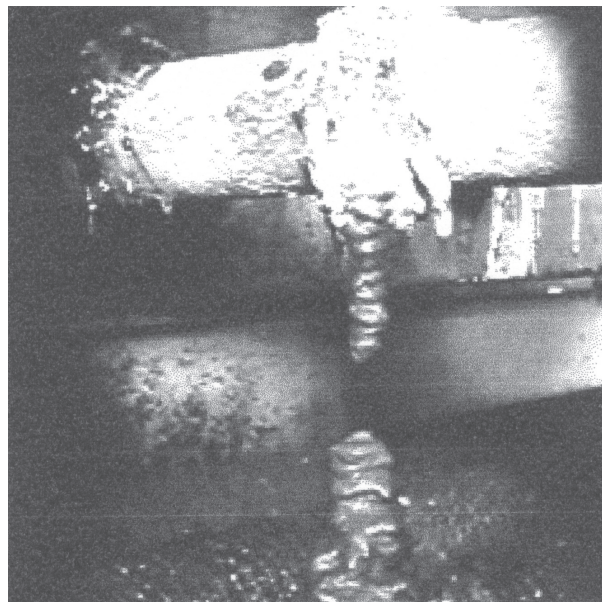
Figure 10-41. Plugged economizer, firing waste fuel
