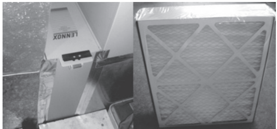
Figure 5-42. Ken's home air filter box and filter
