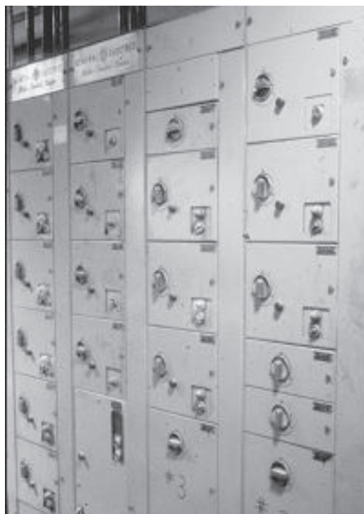
Figure 1-11. Motor control center
