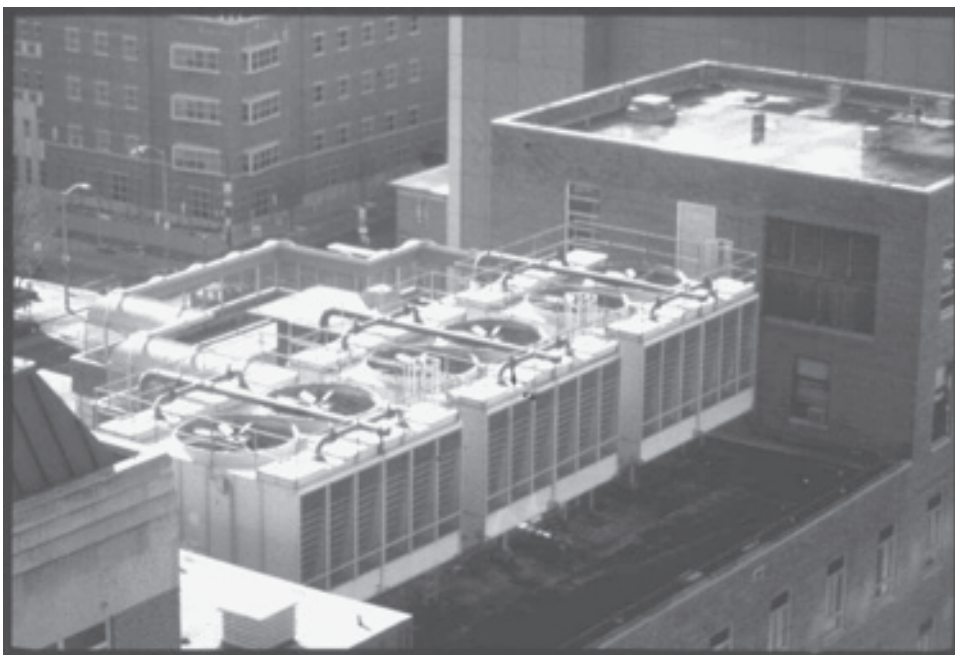
Figure 5-37. Cross flow cooling towers
