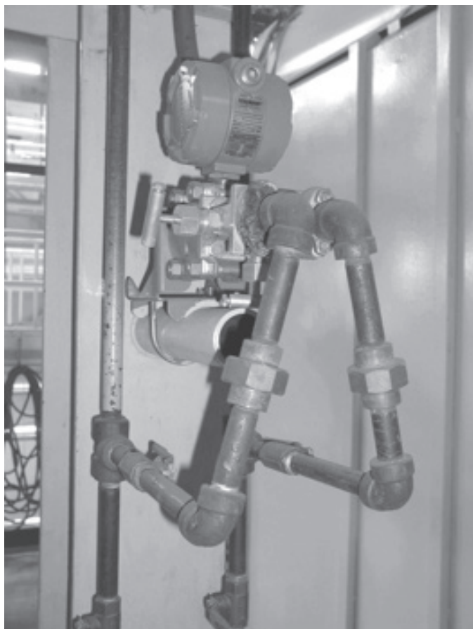
Figure 11-40. Proper transmitter installation
