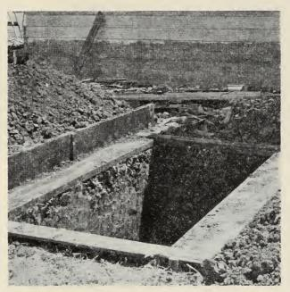
Fig. 4.—The  $2 \times 10$  inch planks laid about the hole are later used as baffie boards.
