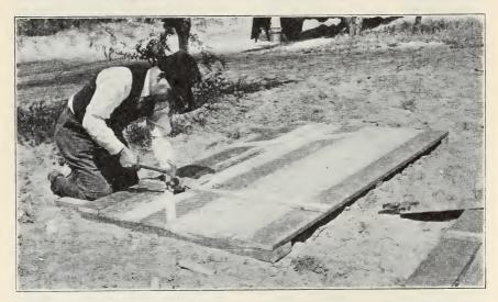
Fig. 8.—Nail the  $1 \times 2$  inch baffie cleats firmly in position after trimming the side-wall sheathing.
