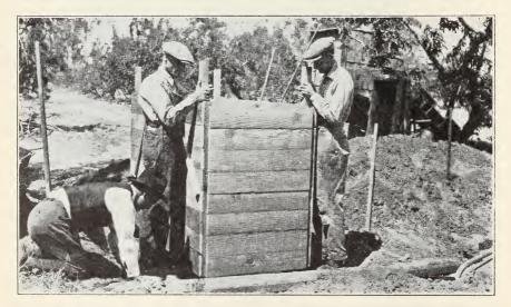
Fig. 11.—The completed form ready to be lowered into the hole.
