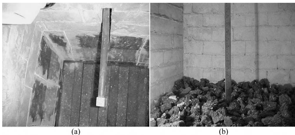
Figure 14.12: Inside view of a radioactive waste incinerator: (a) fire grates, (b) post-combustion chamber filled with silicon carbide (authors' photos).
