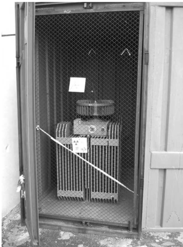
Figure 10.3: A view of a spent RTG in a transport container (authors' photo).
