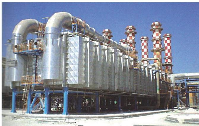
**Figure 6.8** (A) Principle of operation of MED technique with vertical tubes. (B) Industrial conventional installation of MED technique. It produces  $272,520 \text{ m}^3 \text{ day}^{-1}$  desalinated water from seawater with salinity of 42–46‰ (installation June 2008, Bahrain, UAE) (IDA Desalination Year Book, 2008–09).
