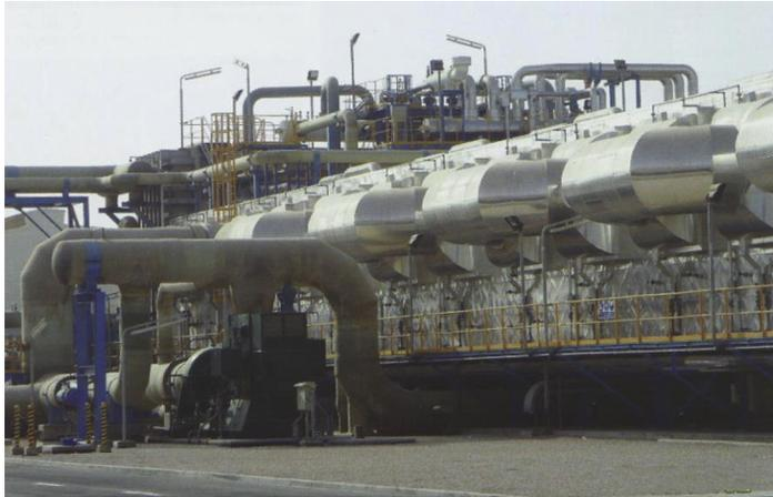
**Figure 6.13** Industrial installation of an MSF system. It comprises four units with a capacity of  $68,130 \text{ m}^3 \text{ day}^{-1}$  each. (Installation June 2008 in Qatar, UAE) (IDA Desalination Year Book, 2008–09).
