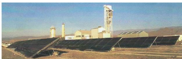
**Figure 6.24** The hybrid desalination system “AQUASOL” with solar system, at Plataforma solar de Almería, Spain (Alarcón et al., 2005).
