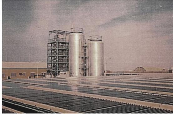
**Figure 6.22** The MES installation and the evacuated tube solar collector field installed in Abu Dhabi (El-Nashar, eolss).
