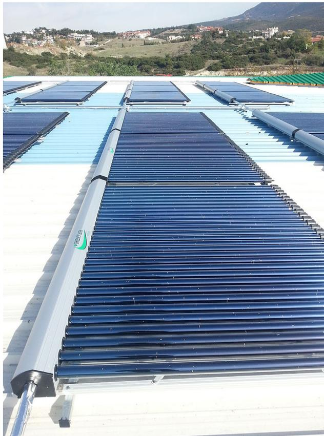
Figure 6.1 Evacuated tube collectors field.
