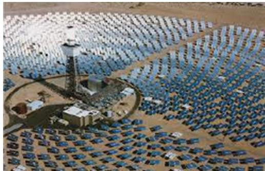
**Figure 6.5** Photograph of the first installed tower system with 1818 heliostats, capacity of 10 MW. The installation is in Barstow, California, USA (Skinrood, 1982).
