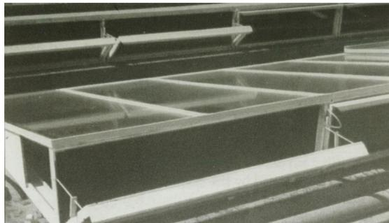
**Figure 3.2** Movable back glass wall for maintenance and cleaning the stills of solar distillation plant in Porto Santo, Madeira, Portugal. *Photograph by E. Delyiannis.*
