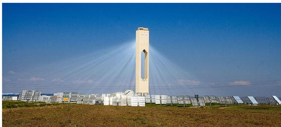
**Figure 6.6** Central tower system with heliostat mirrors. Pictorial view of the first commercial European and international installation (2008). The system is located at Seville, Spain, and produces 11 MW electrical power (Anonymous, 2008).
