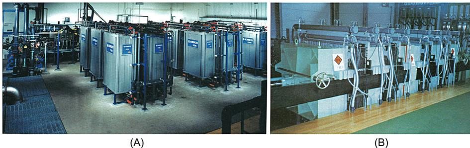
**Figure 1.7** Two electrodesalination installations: (A) The Ionics Inc., Watertown, MA, USA (Ionics Inc., 2002), and (B) electrodesalination cells designed by Ashahi Chemical Industry Com, Japan (Hamada, 1992).
