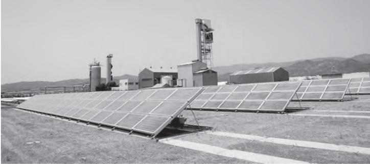
Figure 5. 500 m<sup>2</sup> stationary CPC AQUASOL solar collector field.
