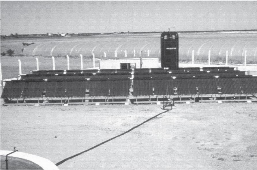
*Figure 1.* Solar desalination plant with single effect process using heat pipes collectors in Hazeg (Tunisia).
