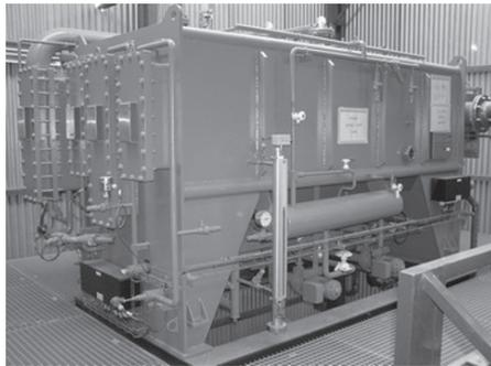
Figure 7. The new double-effect absorption heat pump installed at the PSA.
