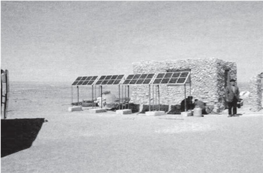
*Figure 2.* Solar batteries for experimental device installed in Aral Sea Region.
