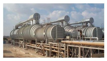
**Figure 2.56** MED - TVC plant with 3 units each 13,333 m<sup>3</sup>/d / Tobruk, Libya (by courtesy of SIDEM (VEOLIA Water Systems) [14].
