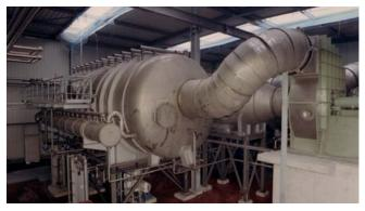
**Figure 2.37** Flow sheet and picture of an evaporation plant with mechanical vapour compression (by courtesy of VA TECH WABAG GmbH).
