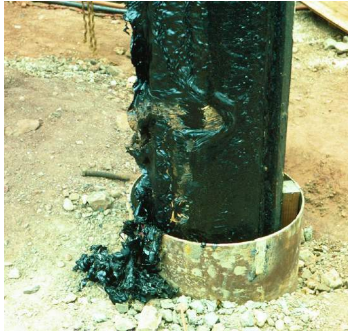
Fig. 7.34 View of a bitumen-coated pile driven through a protective casing The left side of the pile was the pile underside in storage
