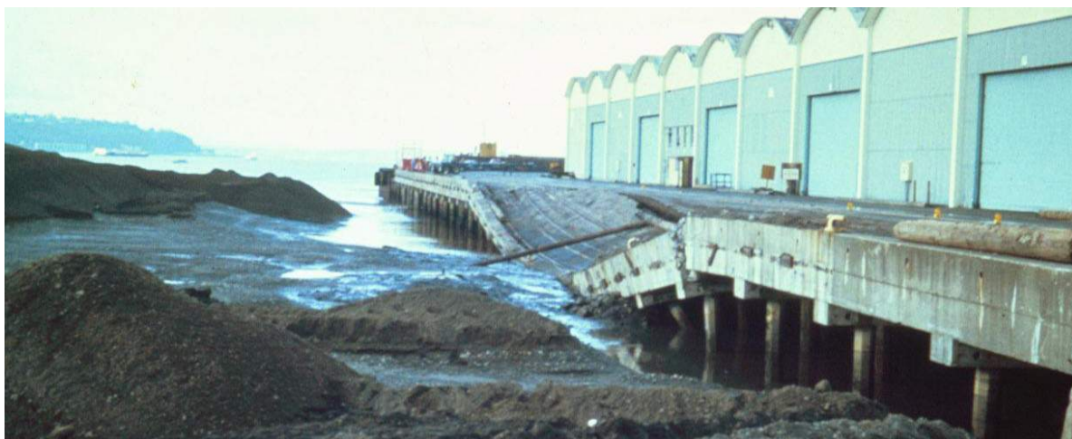
Fig. 7.35 View of the consequence of a hydraulic fill of fine silt flowing against 24-inch piles
