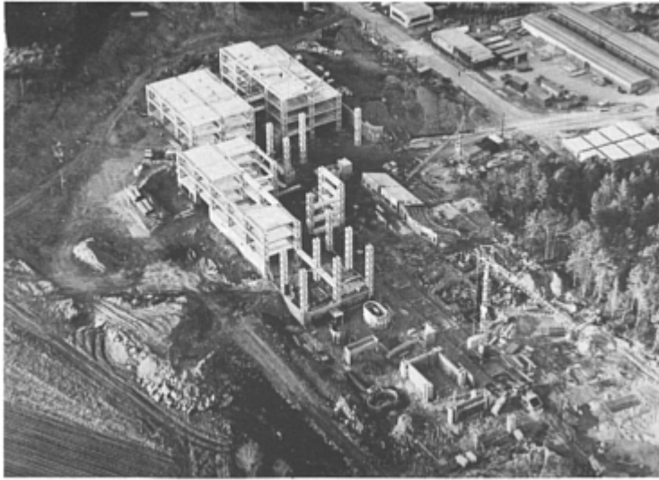
The construction sequence from ground work to frame erection is illustrated in the construction of this university building (Nordlanske Spenbetong AS)
