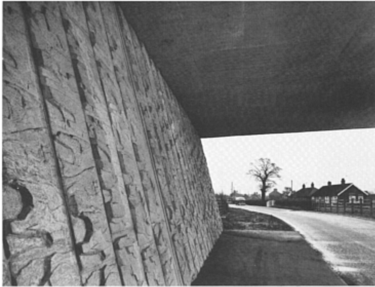
Re-use of formwork—the grp formers used in casting the textured panels illustrated had previously been used on a major road construction (Durham County Council)
