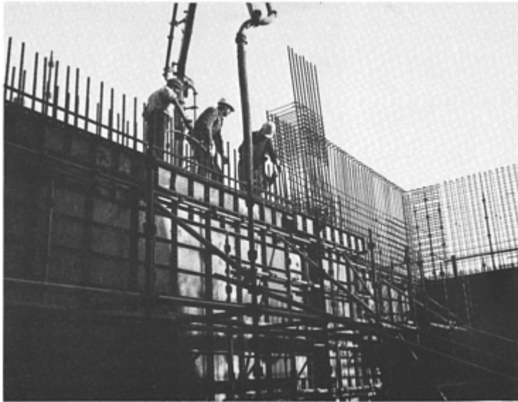
Concreting proceeds around the previously fixed reinforcing steel. Formwork and reinforcement should be considered jointly when planning the construction
