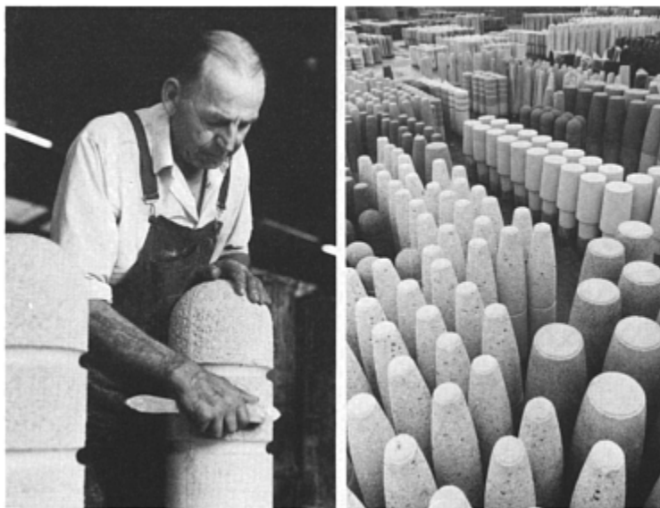
The use of a retarder to produce an attractive finish and improve weathering characteristics of concrete products (Marshall Mono Ltd)
