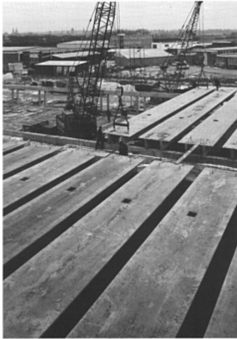
The use of large span double-tee beams reduces the need for falsework and formwork (Dow-Mac Concrete Ltd)
