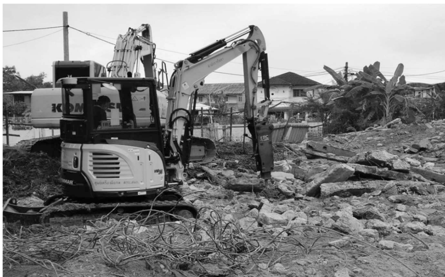
FIGURE 1.5 Demolition of concrete waste from existing foundation concrete structure.
