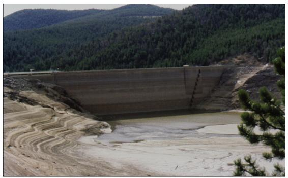
Figure 42.—The downstream face of Barker Dam, near Boulder, Colorado, was resurfaced with prepacked aggregate.
