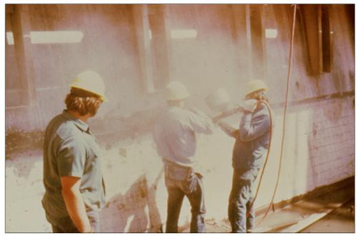
Figure 40.—A small size pneumatic gun can be used to apply portland cement mortar. Regular shotcreting equipment would be too large for this application.
