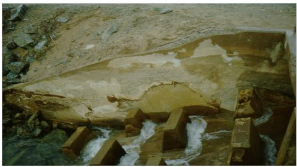
Figure 29.—Concrete damage caused by chloride-induced corrosion of reinforcing steel.
