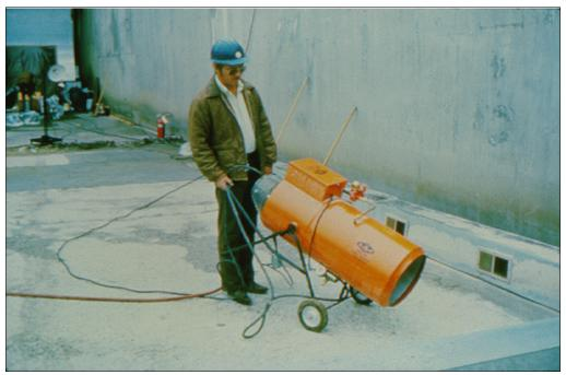
Figure 49.—A gas-fired forced air heater is being used to heat concrete prior to application of epoxy mortar.
