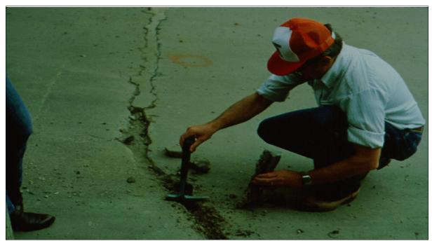
Figure 35.—Improper crack repair techniques often result in short service life.
