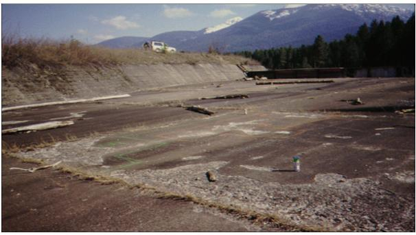
Figure 21.—Freezing and thawing deterioration on spillway concrete.
