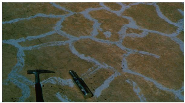
Figure 34.—Inadequate crack repair techniques often result in poor appearance upon completion.
