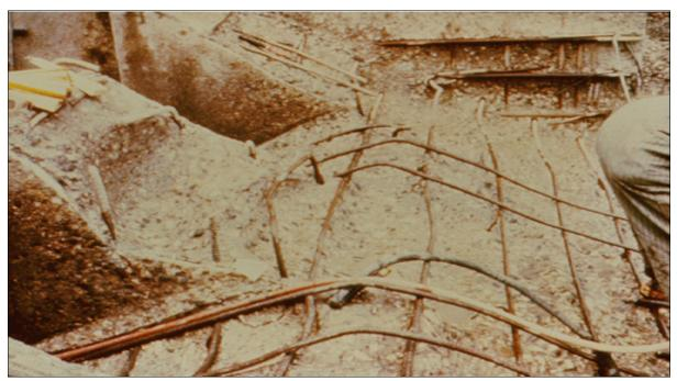
Figure 23.—Abrasion-erosion damage in a concrete stilling basin.
