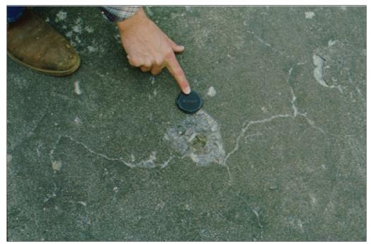
Figure 5.—Absorptive aggregate popout on spillway floor.
