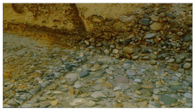
Figure 30.—Concrete deterioration caused by acidic water.
