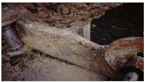
Figure 20.—Freezing and thawing deterioration on small irrigation gate structure.
