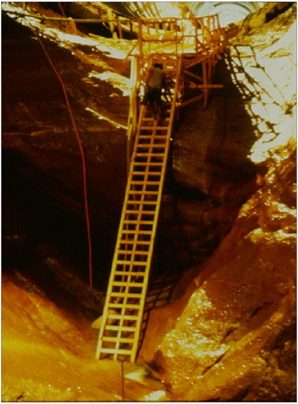
Figure 28.—Extensive cavitation damage to Glen Canyon Dam.
