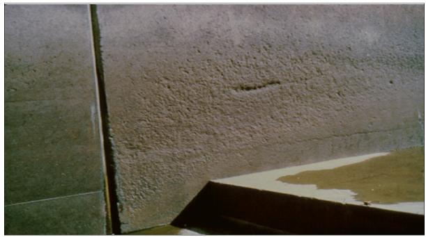
Figure 25.—Early stages of abrasion-erosion damage.
