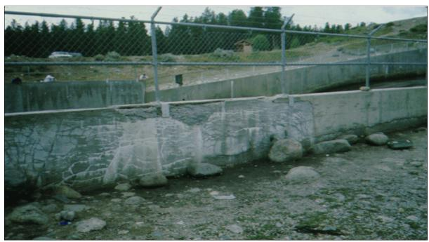
Figure 22.—D-cracking type of freezing and thawing deterioration.
