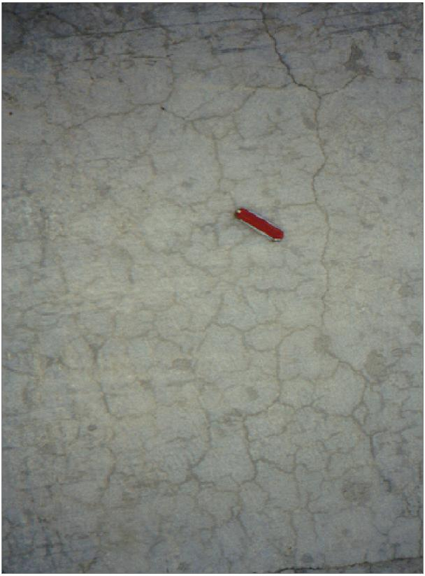
Figure 32.—Typical appearance of drying shrinkage cracking.
