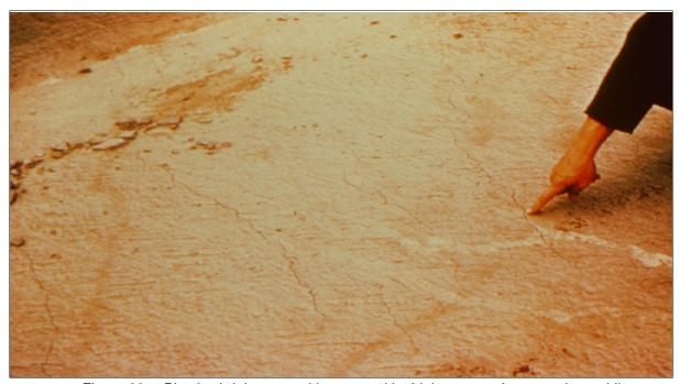
Figure 33.—Plastic shrinkage cracking caused by high evaporative water loss while the concrete was still in a plastic state.
