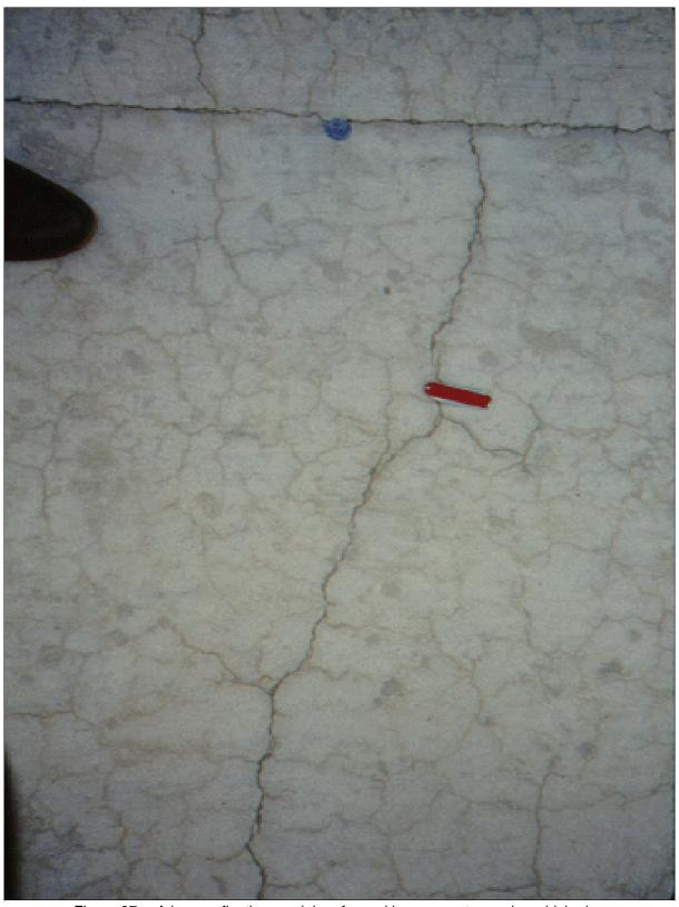
Figure 37.—A large reflective crack has formed in a concrete overlay which also exhibits circular drying shrinkage cracking.
