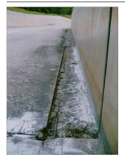
Figure 7.—This concrete damage was found to be a serious threat to the structural integrity of this spillway.
