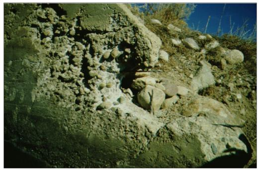
Figure 2.—Deferred maintenance has allowed freezing and thawing deterioration to seriously damage this structure.
