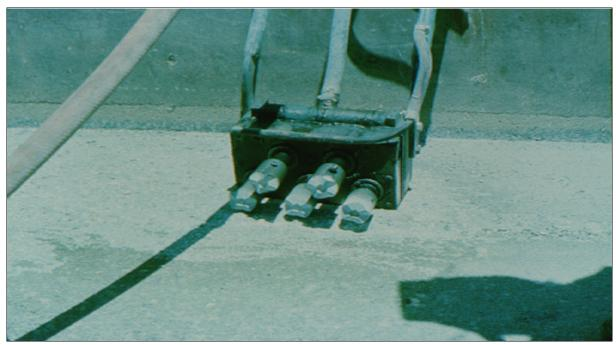
Figure 12.—Multiple bits on the head of a scrabbler pound and pulverize the concrete surface during the removal process.
