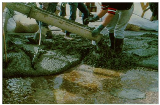
Figure 56.—The placement techniques for epoxy-bonded concrete are essentially the same as for conventional concrete.
