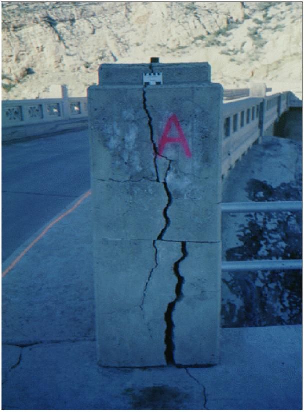
Figure 19.—Severe cracking caused by alkali-aggregate reaction.
