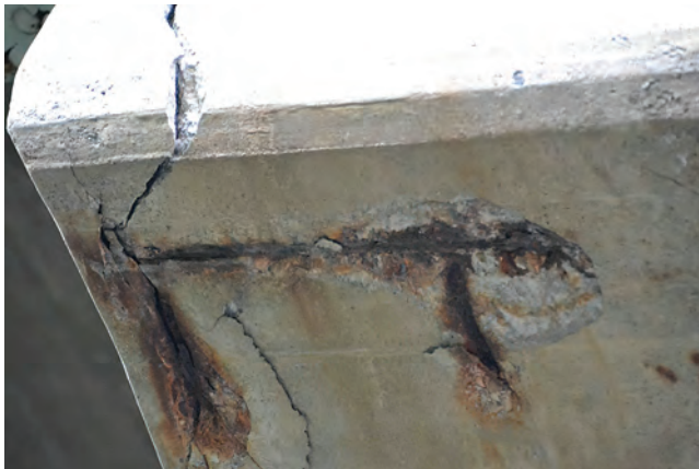
FIGURE 1.24 Steel bar corrosion in concrete structures. (“This is one of a series of 46 pictures, which compares two bridges. The second bridge (picture 46) crosses a canal inside the City of Amsterdam” by Achim Hering.)
