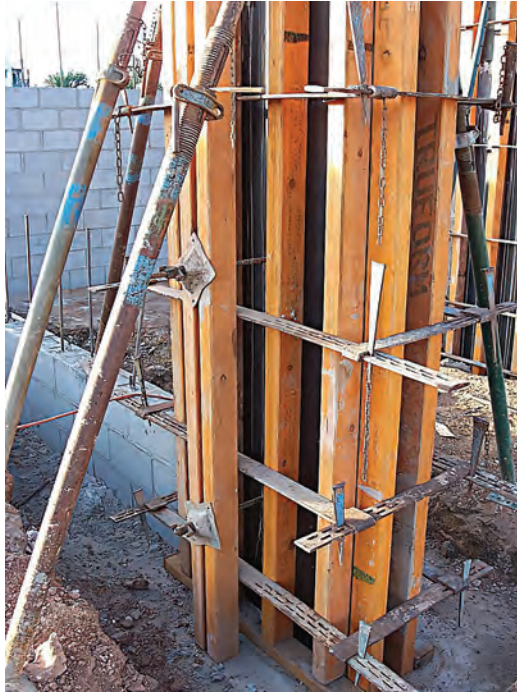
FIGURE 12.15 Wooden forms. (“Column formwork” by Bill Bradley.)
