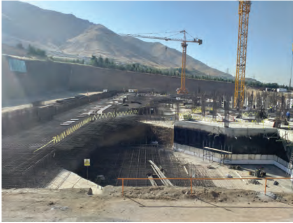
FIGURE 1.8 A mass foundation. (Photograph by the author.)
