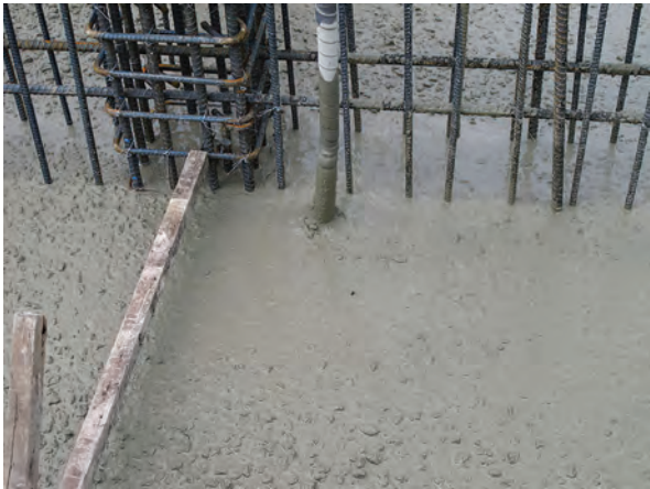
FIGURE 10.24 Concrete vibration. (“Using a vibrating rod to compact and to purge the concrete of any air bubbles”.)
