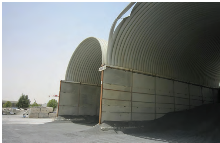
FIGURE 12.5 Shade on the surface of aggregates to control their temperature. (Photograph by the author.)
