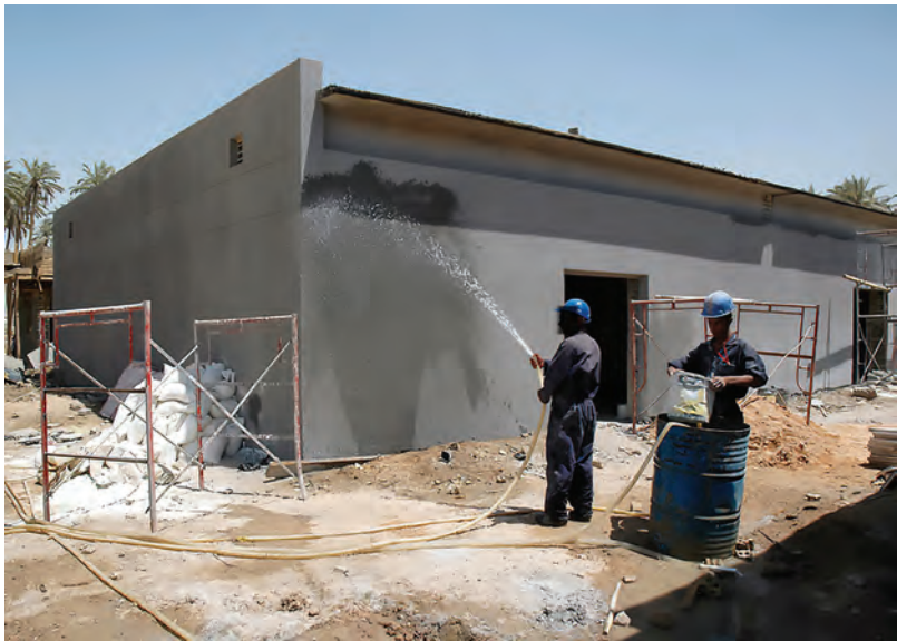
FIGURE 10.28 Water jet curing. (“Iraqi subcontractors use a water base curing process” by Jim Gordon.)
