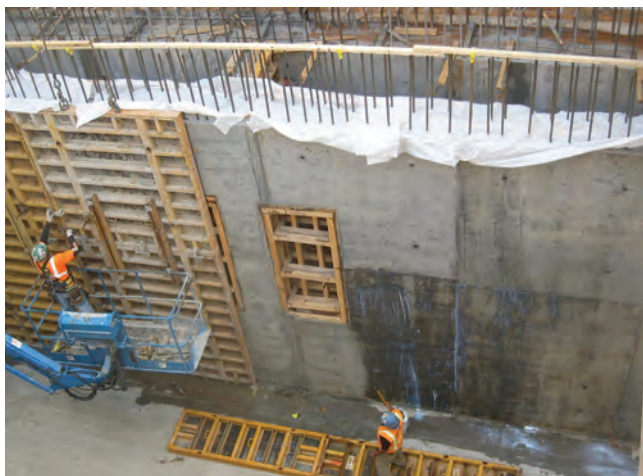
FIGURE 5.25 Application of the curing compound. (“Applying Curing Compound and Stripping the Wall Forms at the Yard Lead Reception Pit” by MTA Construction & Development Mega Projects.)
