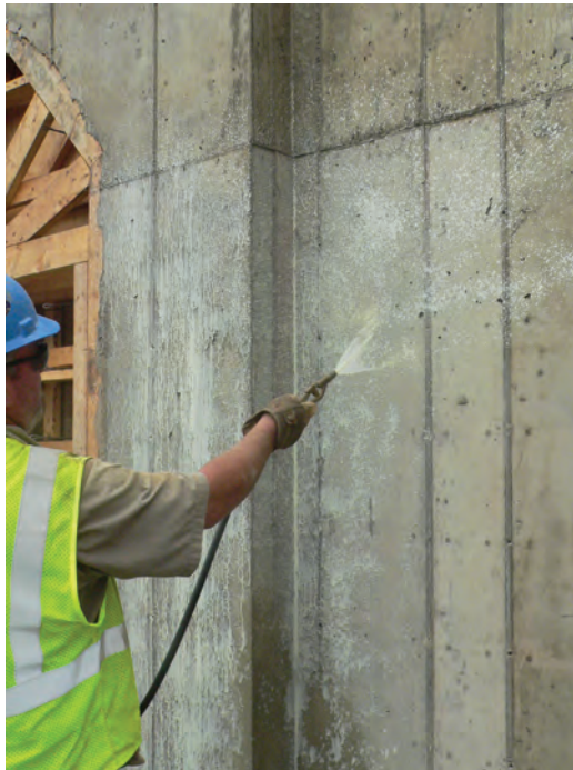
FIGURE 1.10 The implementation of curing compound chemicals. (“Spraying the curing compound” by Robyn McKinley.)
