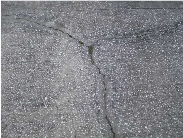
FIGURE 12.9 Concrete cracks that can cause by drying shrinkage and extension due to loading. (“Concrete Cracked” by John Harvey.)
