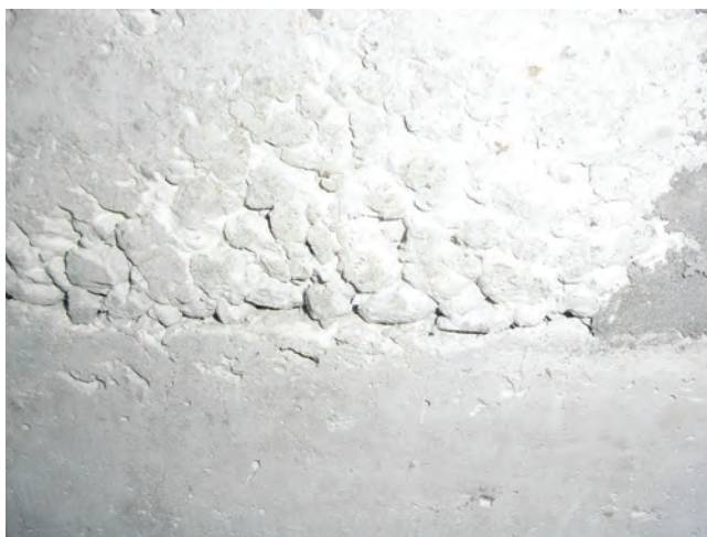
FIGURE 5.26 The result of using a segregated concrete. (“Concrete segregation.”)
