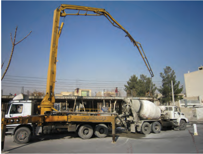
FIGURE 10.20 Concrete pumping. (Photograph by the author.)
