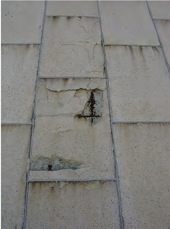
FIGURE 6.3 Corrosion in concrete structures. (“Photograph taken in grounds of Newton Park Technical High School, Port Elizabeth, South Africa”)
