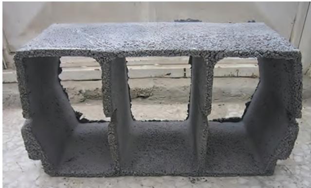
FIGURE 4.15 A type of roof block made with non-structural light weight concrete. (Photograph by the author.)
