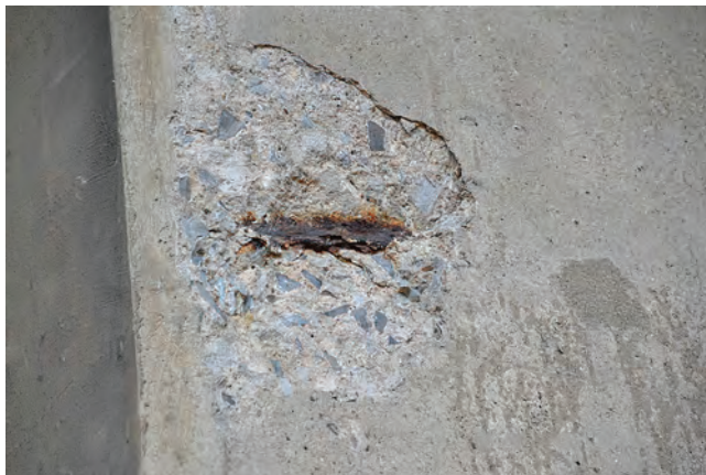
FIGURE 1.25 Corrosion of the steel bars. (“This is one of a series of 46 pictures, which compares two bridges. The first bridge, (pictures 1–45), is part of the Canadian freeway QEW (Queen Elizabeth Way)” by Achim Hering.)
