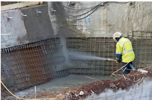
FIGURE 5.3 Applying shotcrete. ("Koln shotcrete application" by Raimond Spekking.)
