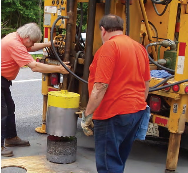
FIGURE 7.23 Huge core taking machine for asphalt and concrete. (“Truck mounted core drill with 14” barrel” by User: Toiyabe used under a Creative Commons Attribution-Share Alike 3.0 Unported license.)
