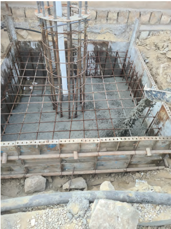
FIGURE 10.23 SCC concrete which is moving through the element. (Photograph by the author.)
