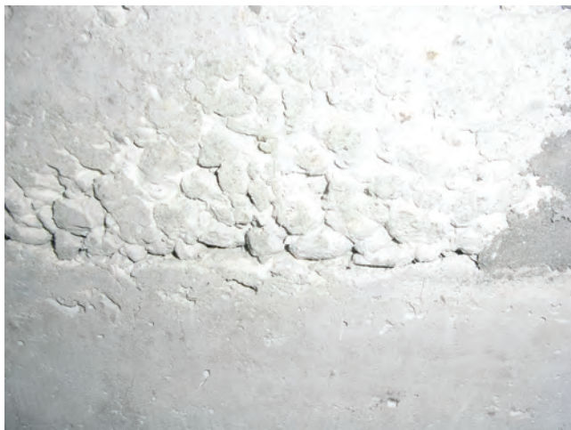
FIGURE 13.2 The result of segregation and bleeding in concrete. (“Concrete segregation”).
