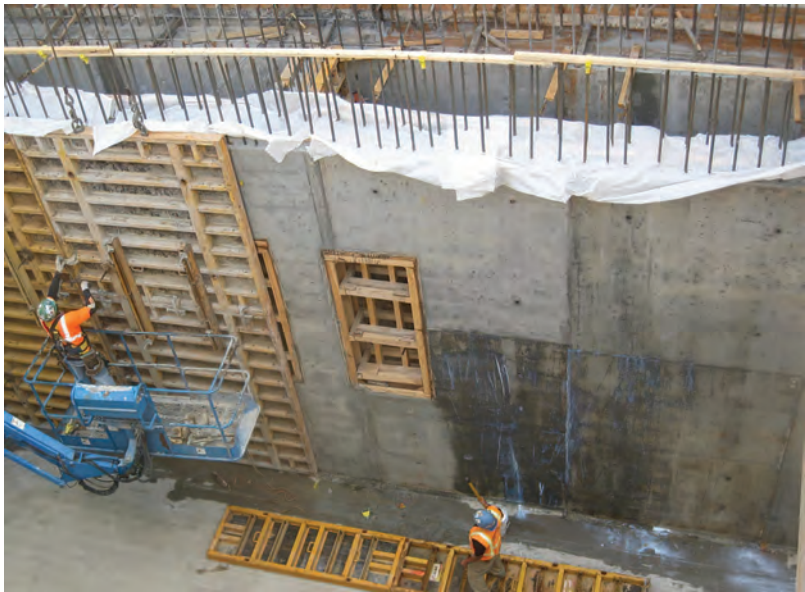
FIGURE 10.27 Using of curing compound for curing of concrete. (“Applying Curing Compound and Stripping the Wall Forms at the Yard Lead Reception Pit” by MTA Construction & Development Mega Projects.)
