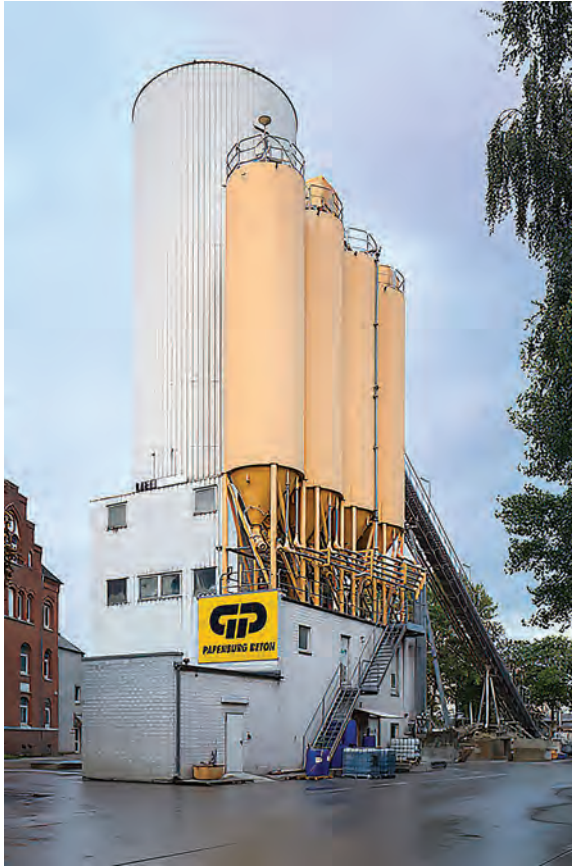
FIGURE 2.29 Cement siloes for the storage of bulk cement. (“Cement silos of Günter Papenburg Beton company” by Christian Schroder.)
