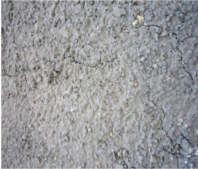
FIGURE 1.5 Cracks on the surface of the concrete. (Photograph by the author.)
