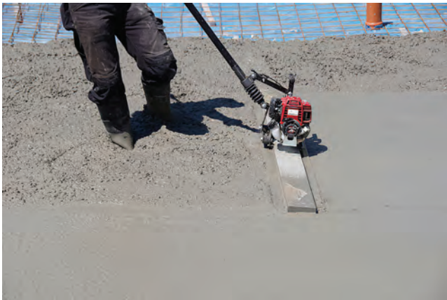
FIGURE 10.25 Electric trowel. (“Flattening of just poured concrete by vibration” by Wouter Hagens.)
