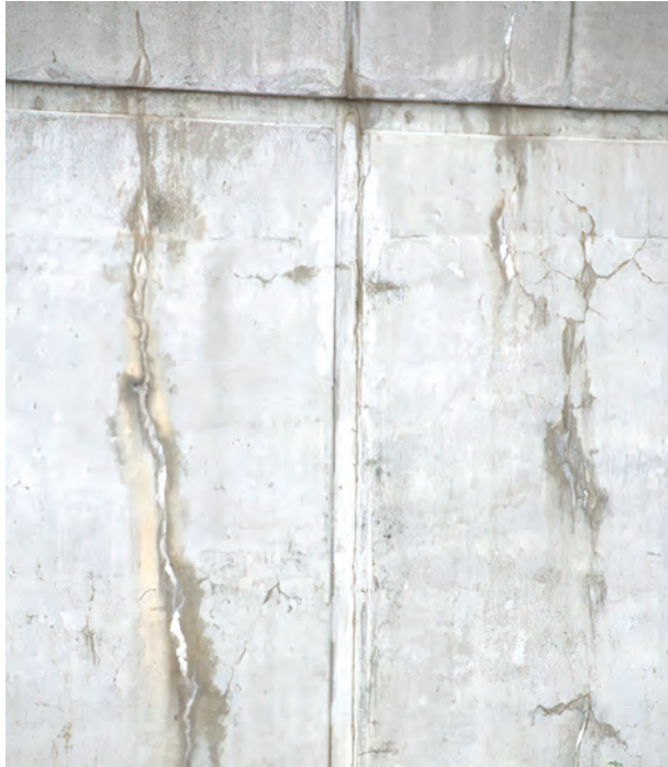
FIGURE 1.23 Alkali aggregate reaction. (“Bc rueckreise 025 swartz bay 2ndary efflorescence alkali silica reactions” by Achim Hering.)
