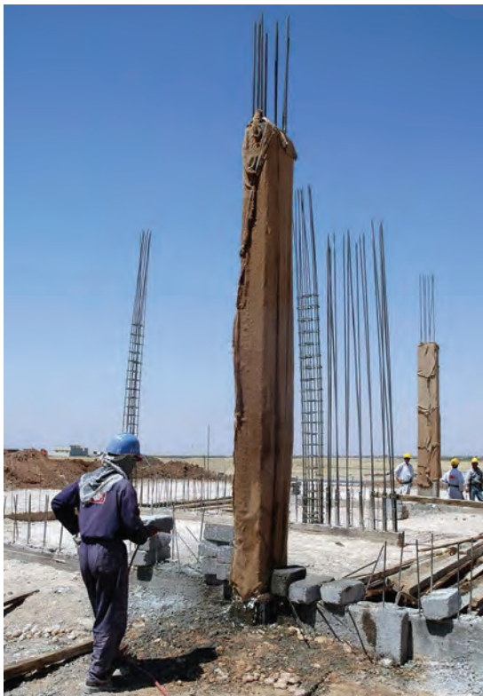
FIGURE 1.11 Water curing of a concrete column. (An Iraqi construction worker” by Jim Gordon.)
