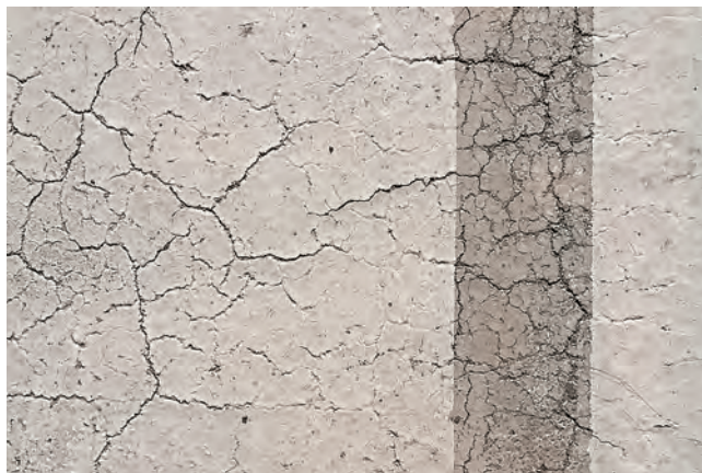
FIGURE 1.27 Cracks on concrete that can be caused by sulfate attack. (“Concrete texture”).
