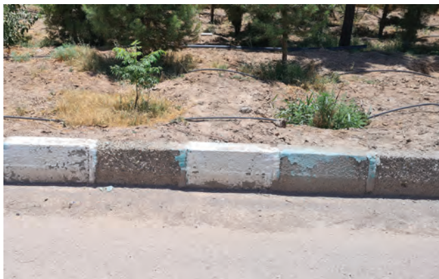
FIGURE 1.28 Freeze-thaw cycles effect on the tables beside a street. (Photograph by the author.)
