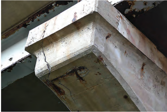
FIGURE 1.26 Corrosion of the steel bars. (“This is one of a series of 46 pictures, which compares two bridges. The second bridge (picture 46) crosses a canal inside the City of Amsterdam” by Achim Hering.)
