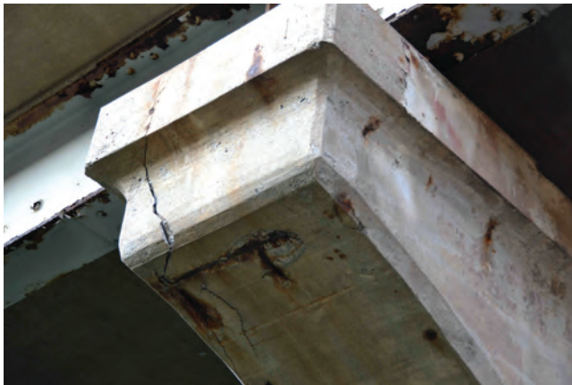
FIGURE 6.2 Corrosion of a concrete bridge. (“The second bridge [picture 46] crosses a canal inside the City of Amsterdam, Netherlands” by Achim Hering.)
