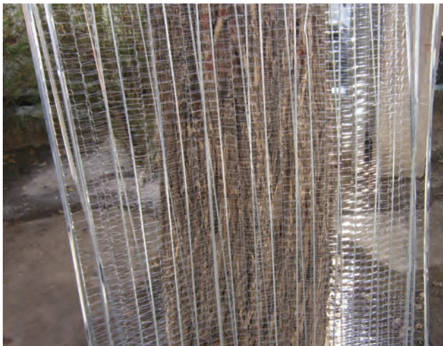
FIGURE 10.26 Expanded metal mesh for dividing the concrete elements. (Photograph by the author.)
