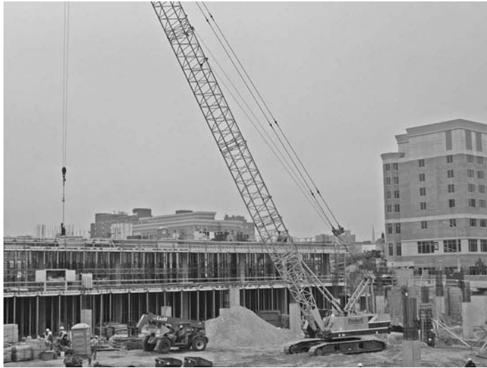
FIGURE 19.20 Crawler crane.
