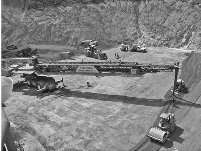
FIGURE 20.1 Placing RCC with 110 lb of cement and 54 lb of fly ash per cubic yard using a 24-in. conveyor at Rompepicos Dam, Mexico. (Photograph courtesy of Ernest K. Schrader.)
