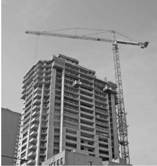
FIGURE 19.9 Top-slewing saddle-jib tower crane.
