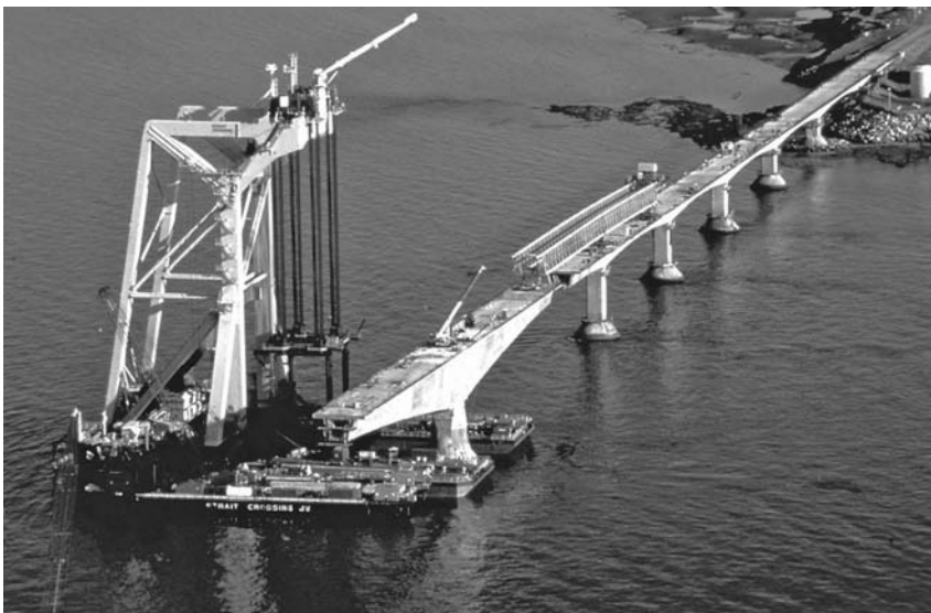
FIGURE 11.41 Prestressed concrete girders being erected at Prince Edward Island Bridge in eastern Canada.
