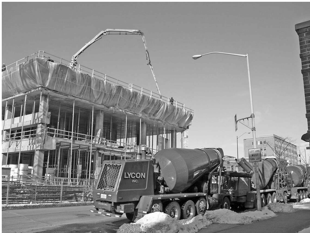
FIGURE 19.4 Truckmixers lined up on the street, awaiting their turn to enter the restricted site and position themselves at the concrete pump.
