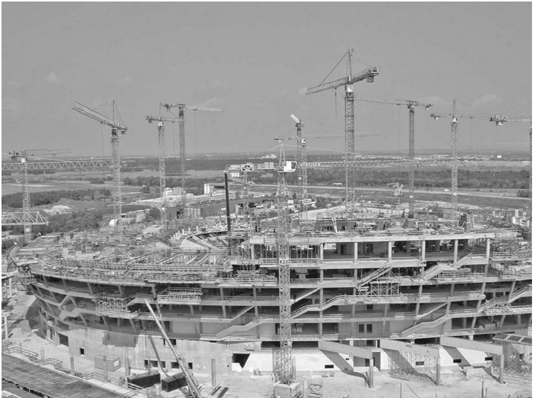
The construction of the Allianz Arena, a 70,000-capacity stadium in Munich, Germany, makes a fine example of a multi-crane site. Nearly 20 tower cranes, as well as several mobile cranes, were in use when this photograph was taken in September of 2003. (Photograph courtesy of Israel Mizrahi, Israel.)
