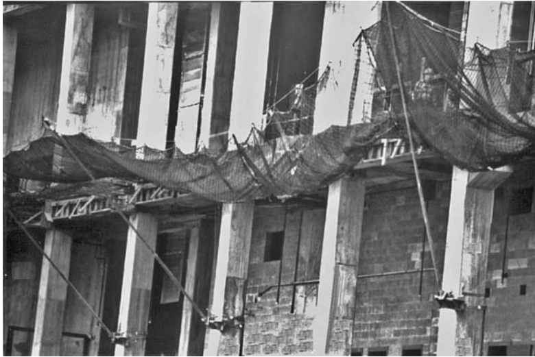
FIGURE 7.23 Fall-protection nets.
