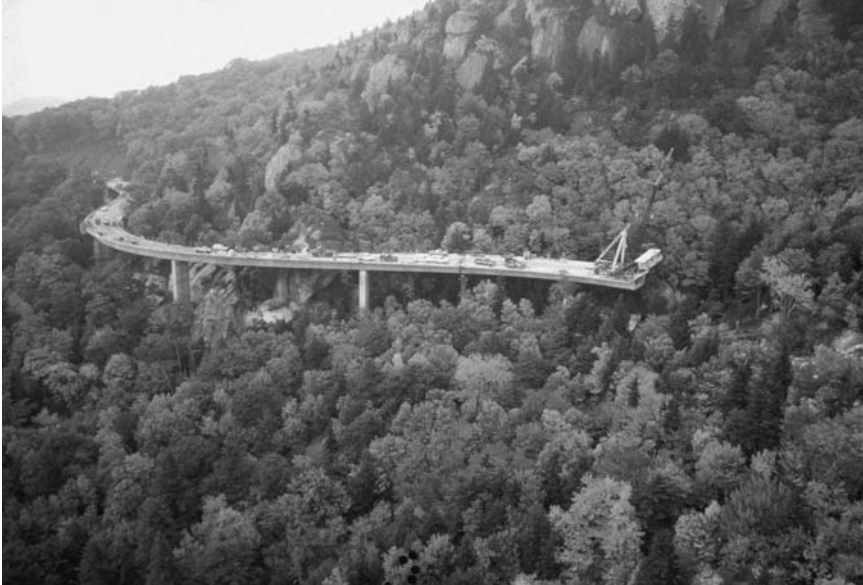
FIGURE 29.11 North Carolina's Blue Ridge Parkway Viaduct was built from the top to protect the sensitive environment so the mountain's owner would allow construction of this important link.
