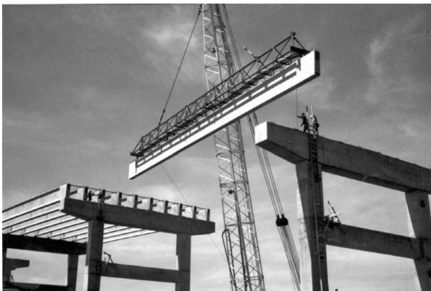
FIGURE 11.31 Erecting precast girder using trussed spreader beam. (From Gerwick, B.C., Jr., Construction of Prestressed Concrete Structures , John Wiley & Sons, New York, 1996. With permission.)
