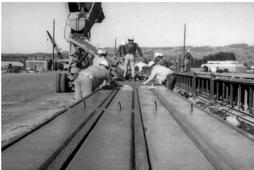
FIGURE 11.22 Concreting and finishing operations.
