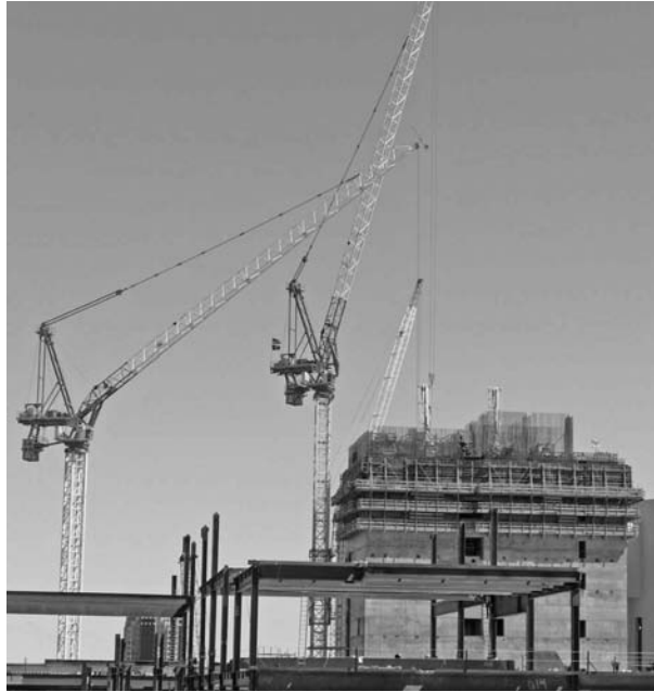
FIGURE 19.14 Top-slewing luffing-jib tower cranes.
