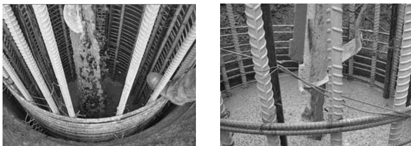
FIGURE 15.10 SCC in drilled shafts.
