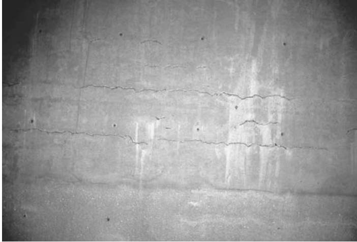
FIGURE 30.37 Concrete wall placed with a superplasticizer in the mixture and no internal or external vibration; settlement lines occurred at all horizontal reinforcing locations.
