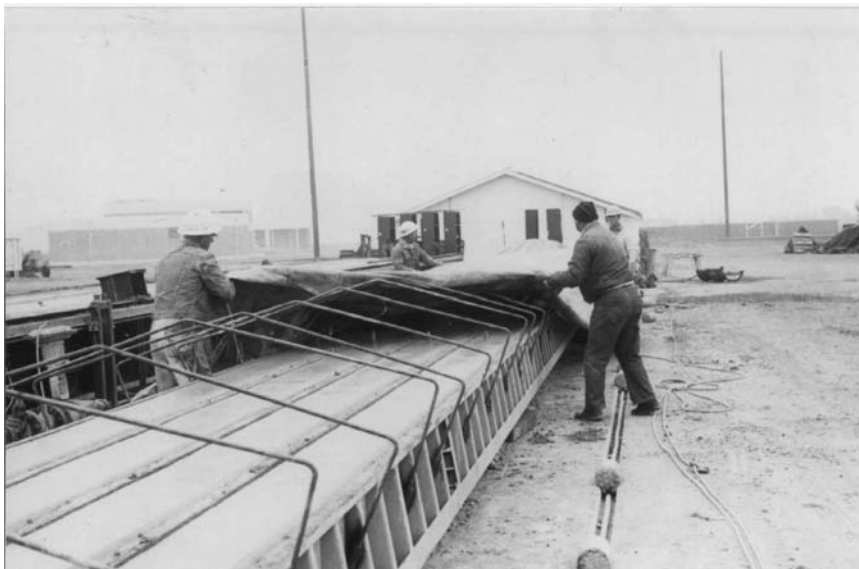
FIGURE 11.3 Spreading rubberized nylon tarpaulins in preparation for steam curing. (From Gerwick, B.C., Jr., Construction of Prestressed Concrete Structures , John Wiley & Sons, New York, 1996. With permission.)
