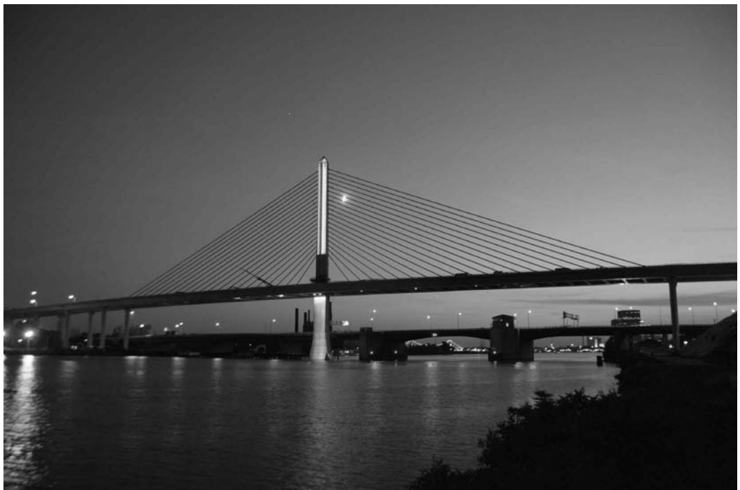
I-280 Veterans' Glass City Skyway Bridge in Toledo, Ohio. Designed by FIGG for the Ohio Department of Transportation. This signature cable-stayed bridge features a pylon with four sides of glass and LED lighting.
