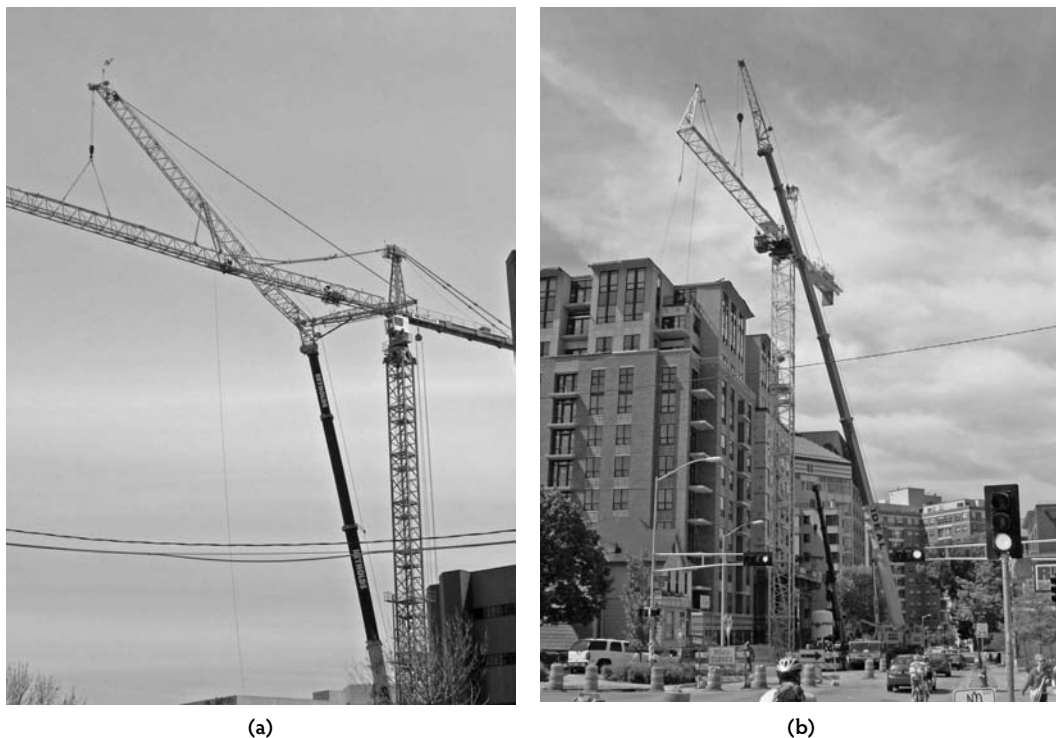
FIGURE 19.15 Erecting and dismantling a top-slewing tower crane using a mobile crane: (a) erecting; (b) dismantling. Note the lane closure and interruption to traffic.
