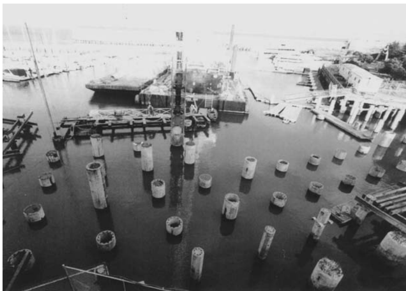
FIGURE 11.49 Pretensioned hollow-core piles driven to support new pier in San Francisco Bay.
