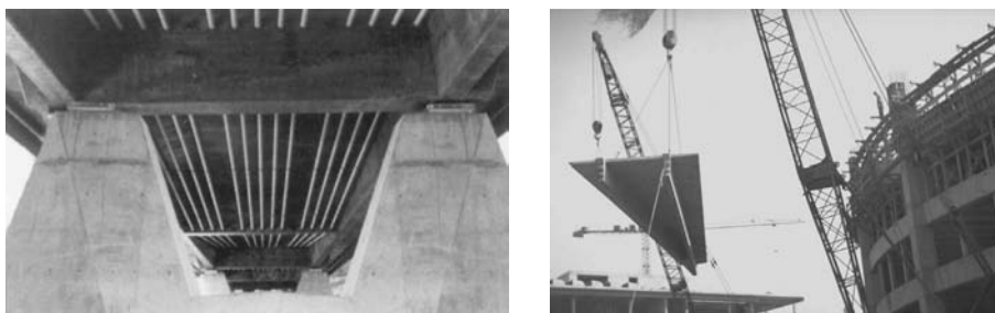
VSL External Post-Tensioning System Components
