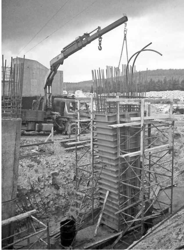
FIGURE 19.25 Knuckle-boom truck loader in form-assembly work.
