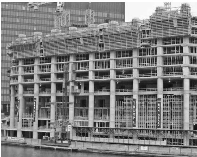
FIGURE 19.30 Crane-independent self-climbing forming system (Trump Tower, Chicago).
