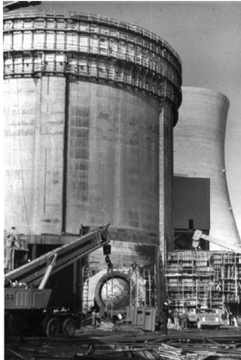
FIGURE 7.3 Large and complex placements require substantial formwork.
