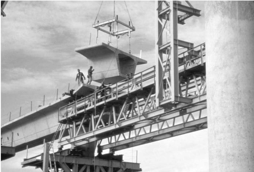
FIGURE 29.15 AirTrain JFK, the light rail system around New York's JFK Airport, was erected utilizing both span-by-span and balanced cantilever construction methods to achieve an aggressive schedule.
