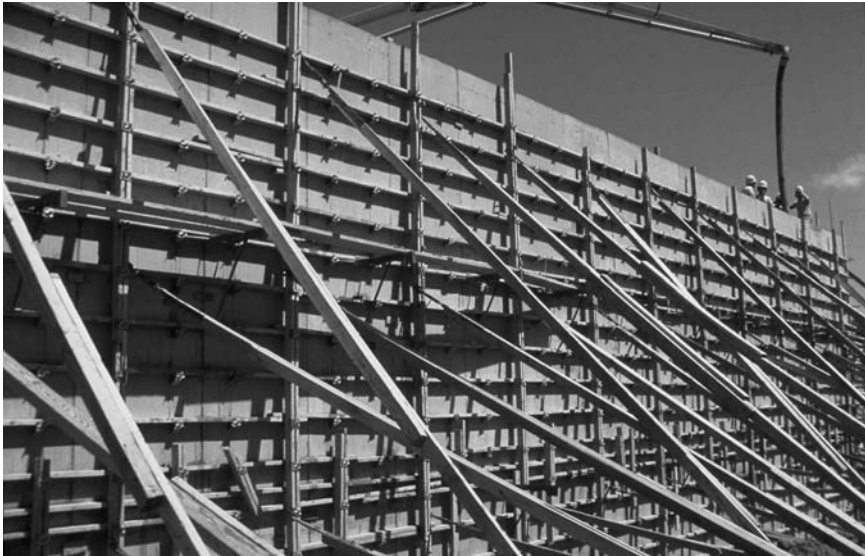
Framework for concrete wall. (Photograph courtesy of Portland Cement Association, Skokie, IL.)
