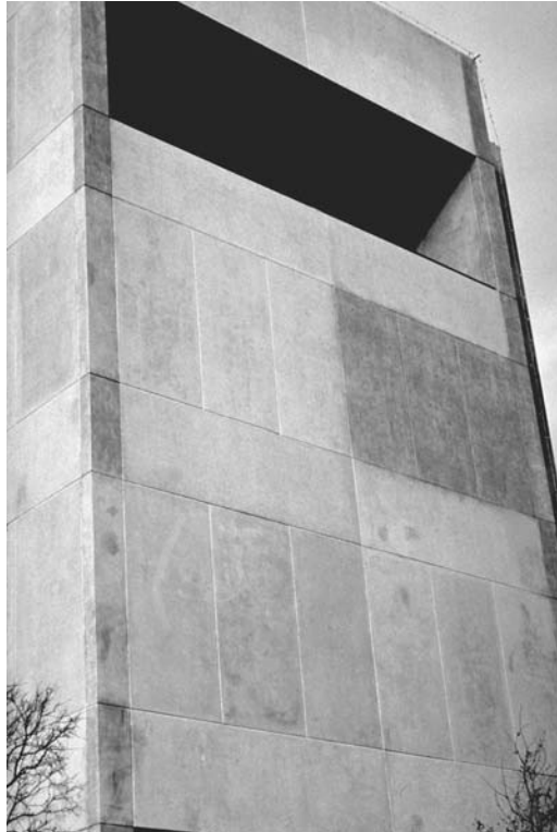
FIGURE 30.11 Wood forms having varying degrees of absorbance as new sections have been added to gang forms.
