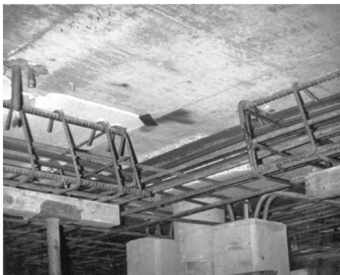
FIGURE 12.34 Tendons installed within a reinforcing cage.
