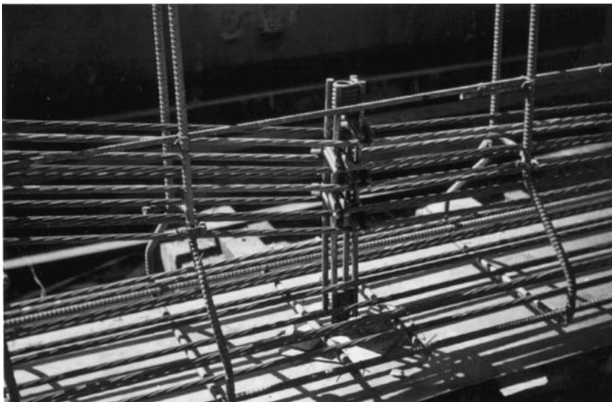
FIGURE 11.23 Deflecting pretensioned strands with special hold-down devices. (Photograph courtesy of Ben C. Gerwick, Inc., San Francisco, CA.)
