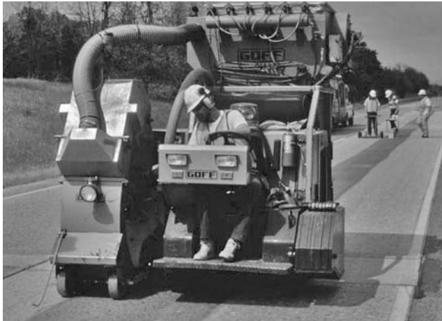
FIGURE 23.2 Shot blast provides for good bond strength by cleaning and texturing the concrete surface.
