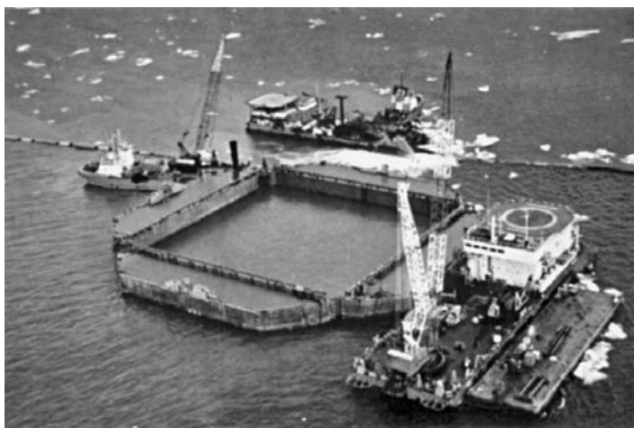
FIGURE 13.21 Concrete retaining-wall caissons. (From Anon., Ocean Industry , 21(8), 32, 1986.)
