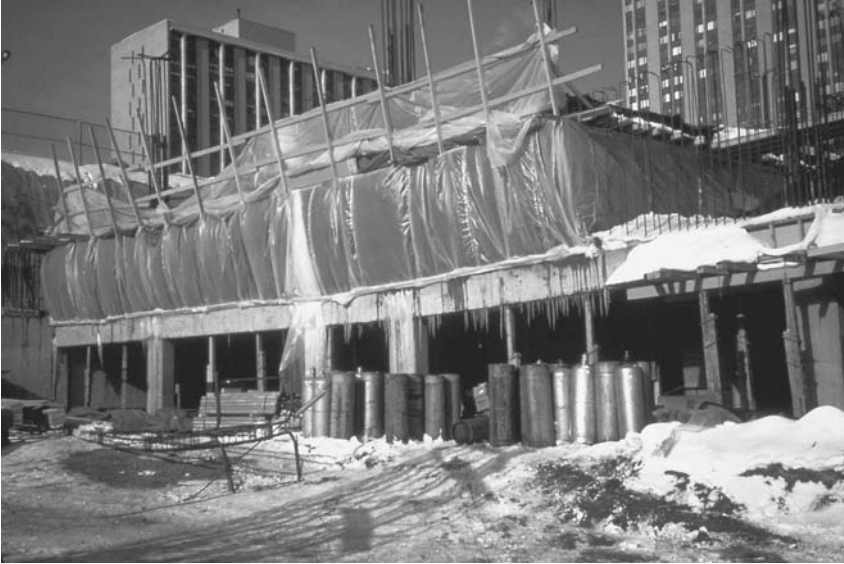
FIGURE 5.27 Cold-weather concreting under suitable preparation conditions. (Figure courtesy of the Portland Cement Association, Skokie, IL.)
