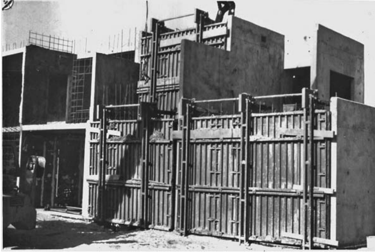
FIGURE 7.1 Formwork serves as a mold to define concrete structure shape.
