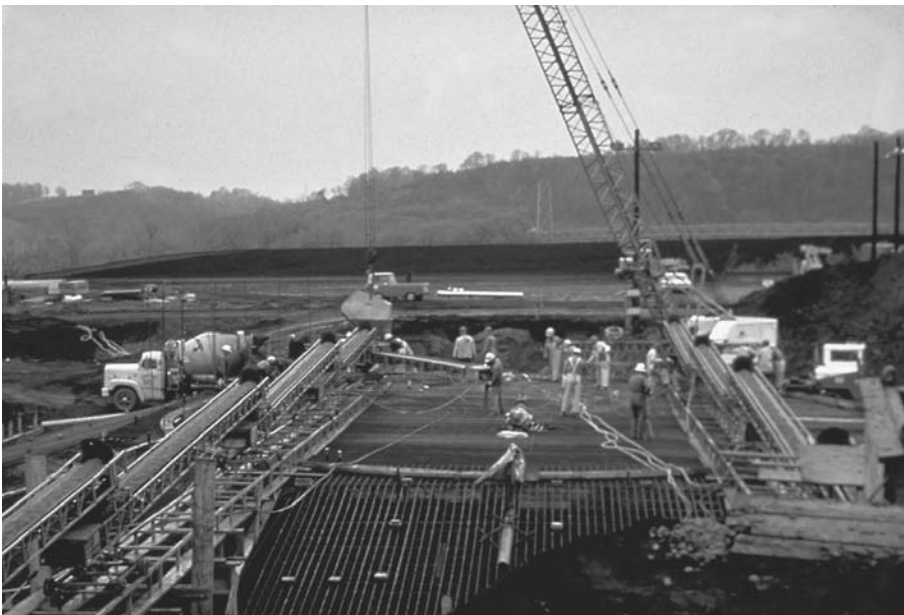
FIGURE 30.30 Conveyors in use at construction site.
