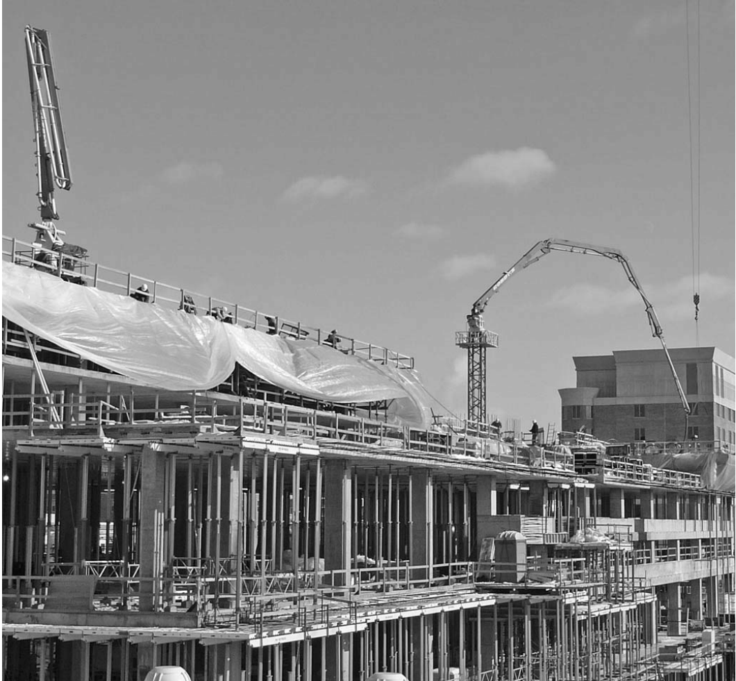
FIGURE 19.7 Climbing placing booms.
