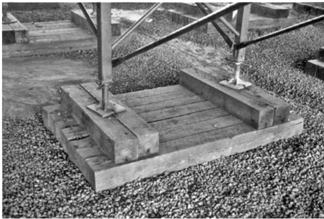
FIGURE 7.36 Wood timber grillage mudsill.
