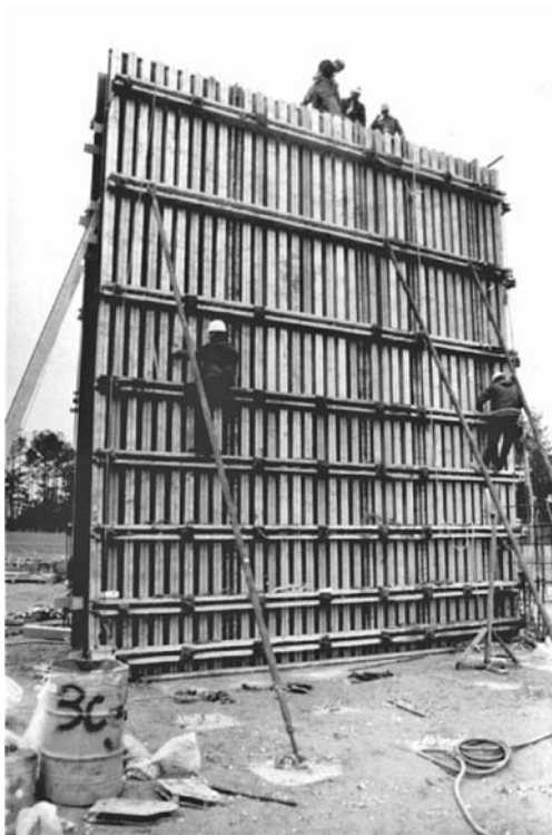
FIGURE 7.25 Preengineered wall form system.
