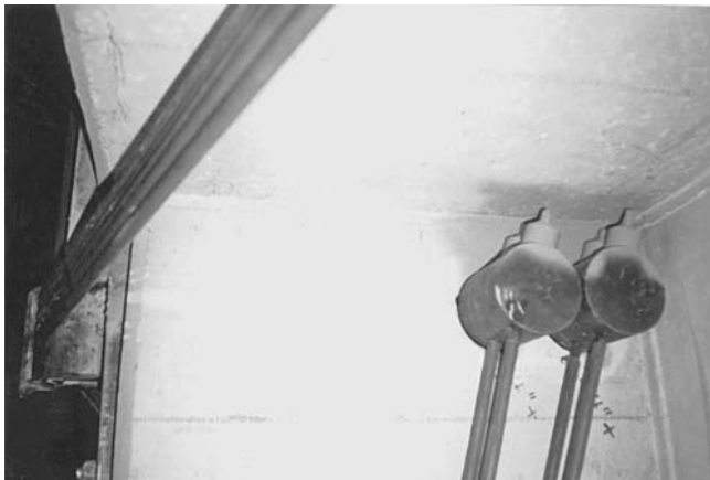
FIGURE 12.26 Alternative connection of external unbonded tendons.
