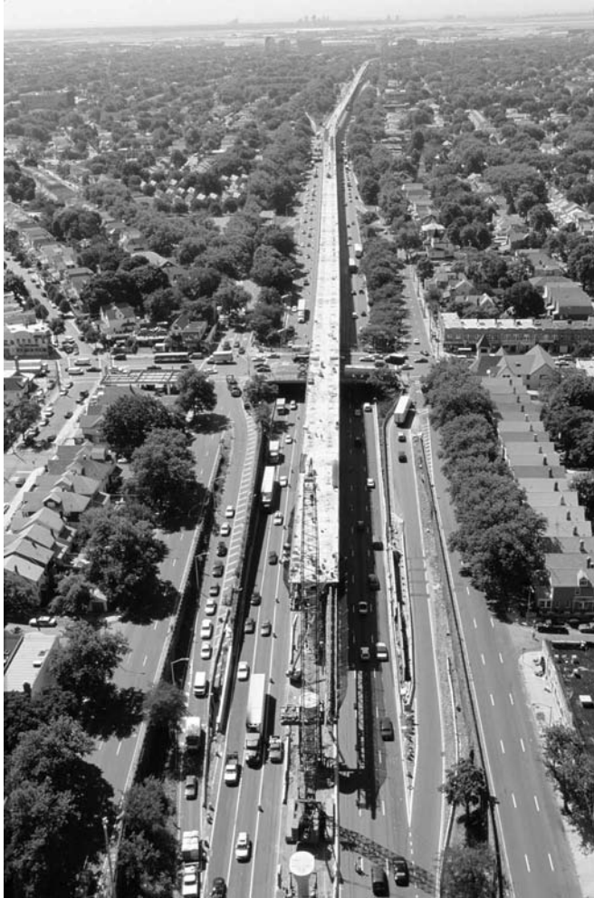
FIGURE 29.19 Span-by-span erection was completed in the median of the Van Wyck Expressway, where over 160,000 vehicles pass each day.
