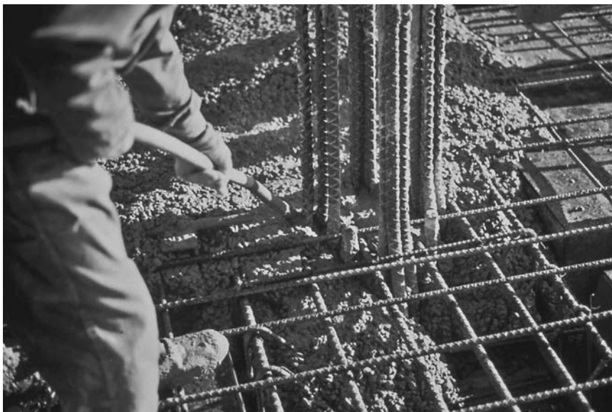
FIGURE 5.8 Proper vibration facilitates concrete placement even in heavily reinforced members. (Figure courtesy of the Portland Cement Association, Skokie, IL.)
