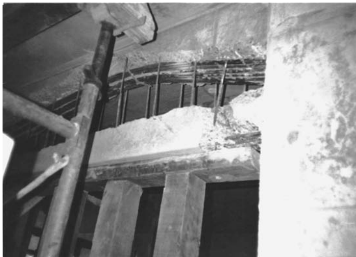
FIGURE 12.22 Misaligned tendon revealed by destructive testing.
