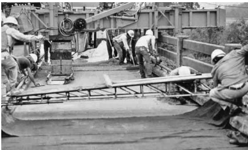
FIGURE 23.10 Wet burlap is placed on the overlay surface as soon as possible to prevent plastic shrinkage cracks.
