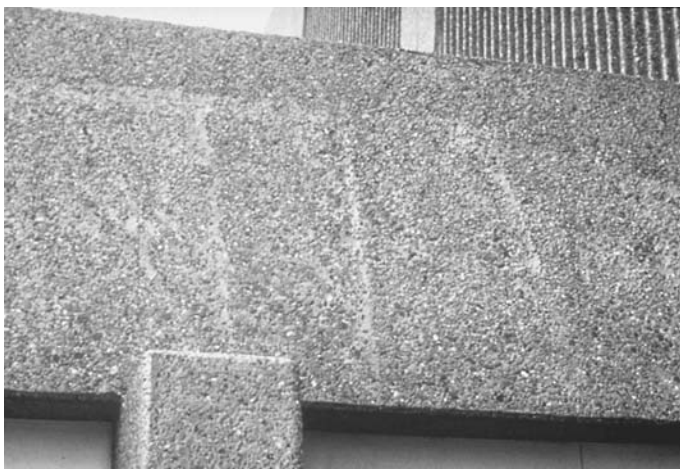
FIGURE 30.36 Grout lines on exposed face of architectural concrete due to an internal vibrator touching the side of the form during concrete consolidation.
