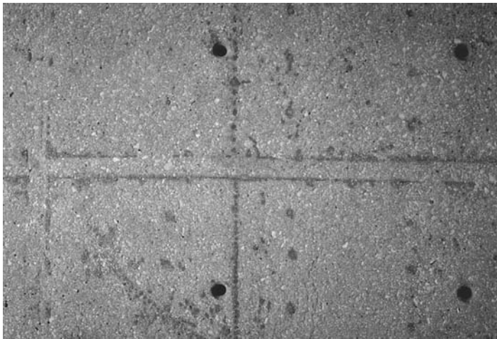
FIGURE 30.13 Moisture leakage at nail holes and at the edges of duct tape used at form butt joints reduce the w/c ratio at the point of migration, resulting in dark areas in the concrete surface.
