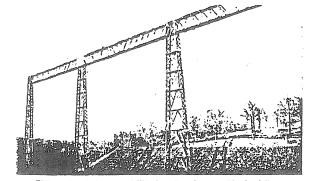
FIG. 3—The University of Illinois radio telescope. The focal line array, 155 feet above the 400-by-600-foot parabolic reflector, is visible below the wooden trues
