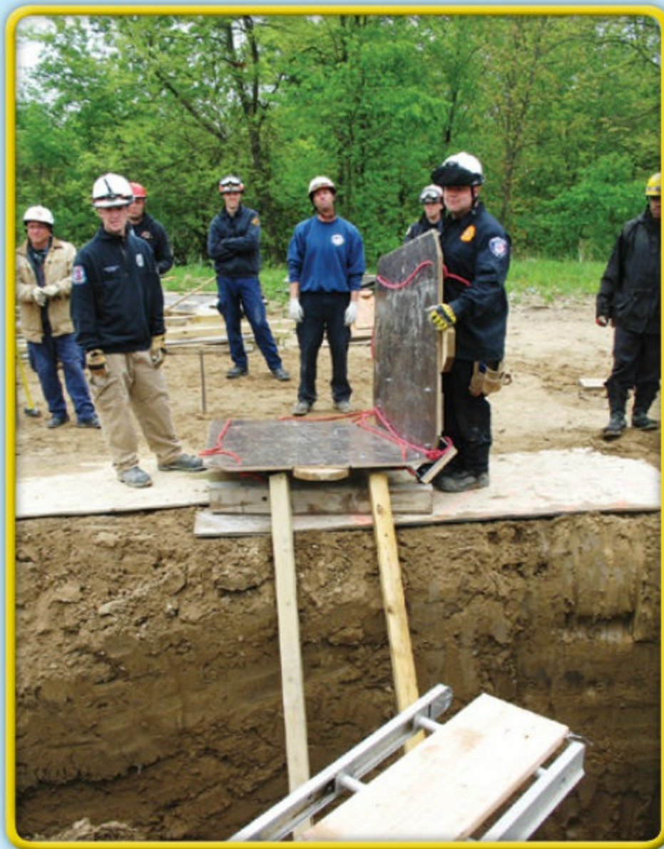
1 Assemble the inside corner panels (bolt on corner brackets) while working on lip protection. Courtesy of Ron Zawlocki
