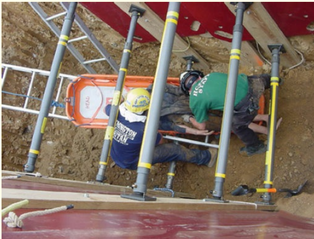
FIGURE 12-15 When deciding on patient packaging devices, consider the limiting factor of the shoring system.
