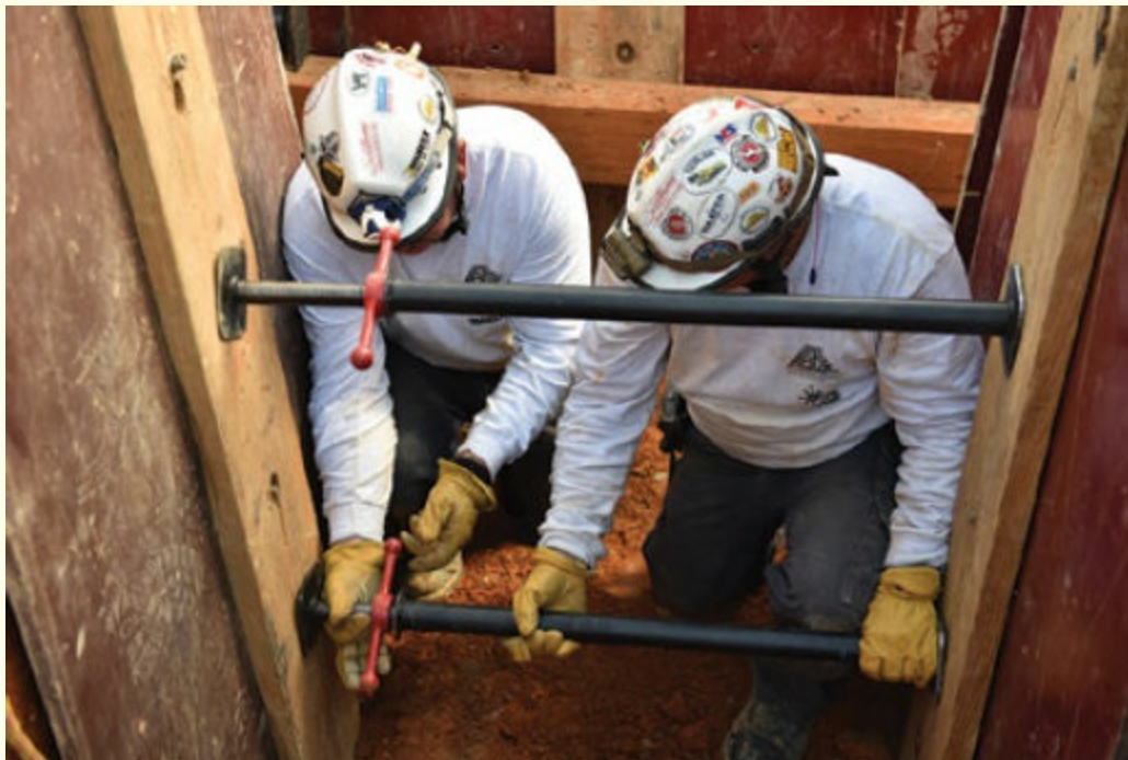
FIGURE 6-14 Screw jacks are very versatile and relatively inexpensive.
