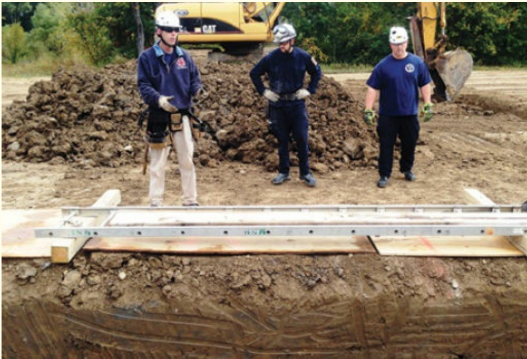
FIGURE 10-2 Fire service ladders with 2 × 12-inch lumber can be used as lip bridge beams and decking. Courtesy of Ron Zawlocki
