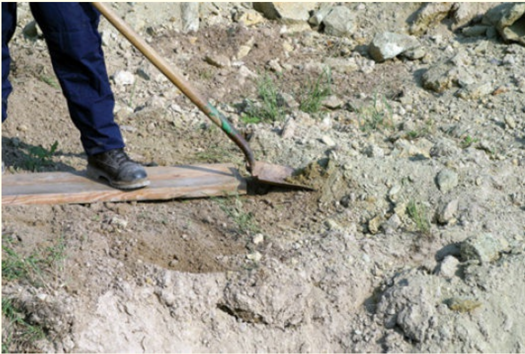
FIGURE 4-13 Rescue personnel should always stand on ground pads while moving the spoil pile. Courtesy of Cecil V. "Buddy" Martinette, Jr.
