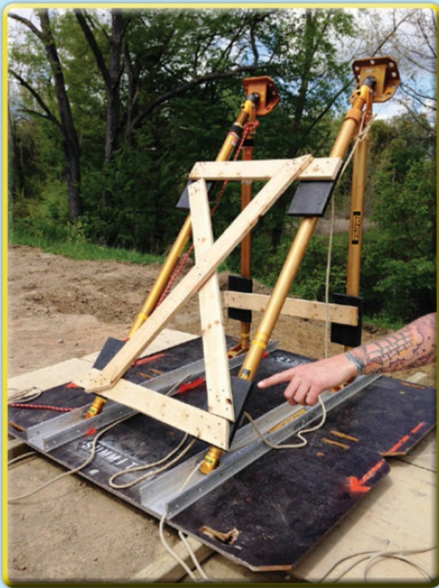
3 Nail 2 × 6-inch bracing to the rakers. Courtesy of Ron Zawlocki
