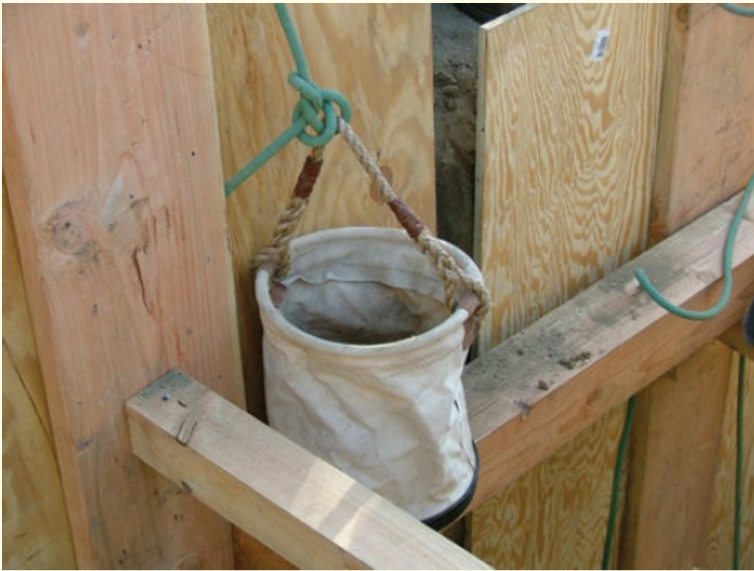
FIGURE 12-7 Dirt bag being used to excavate spoil from a trench.
