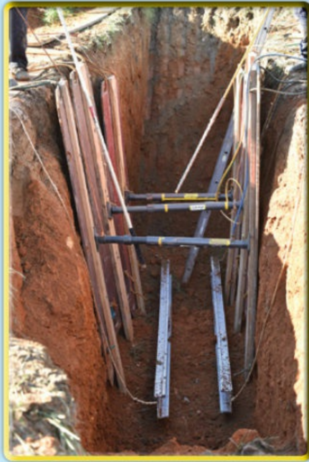
6 Install the middle shores on the outside panels.
