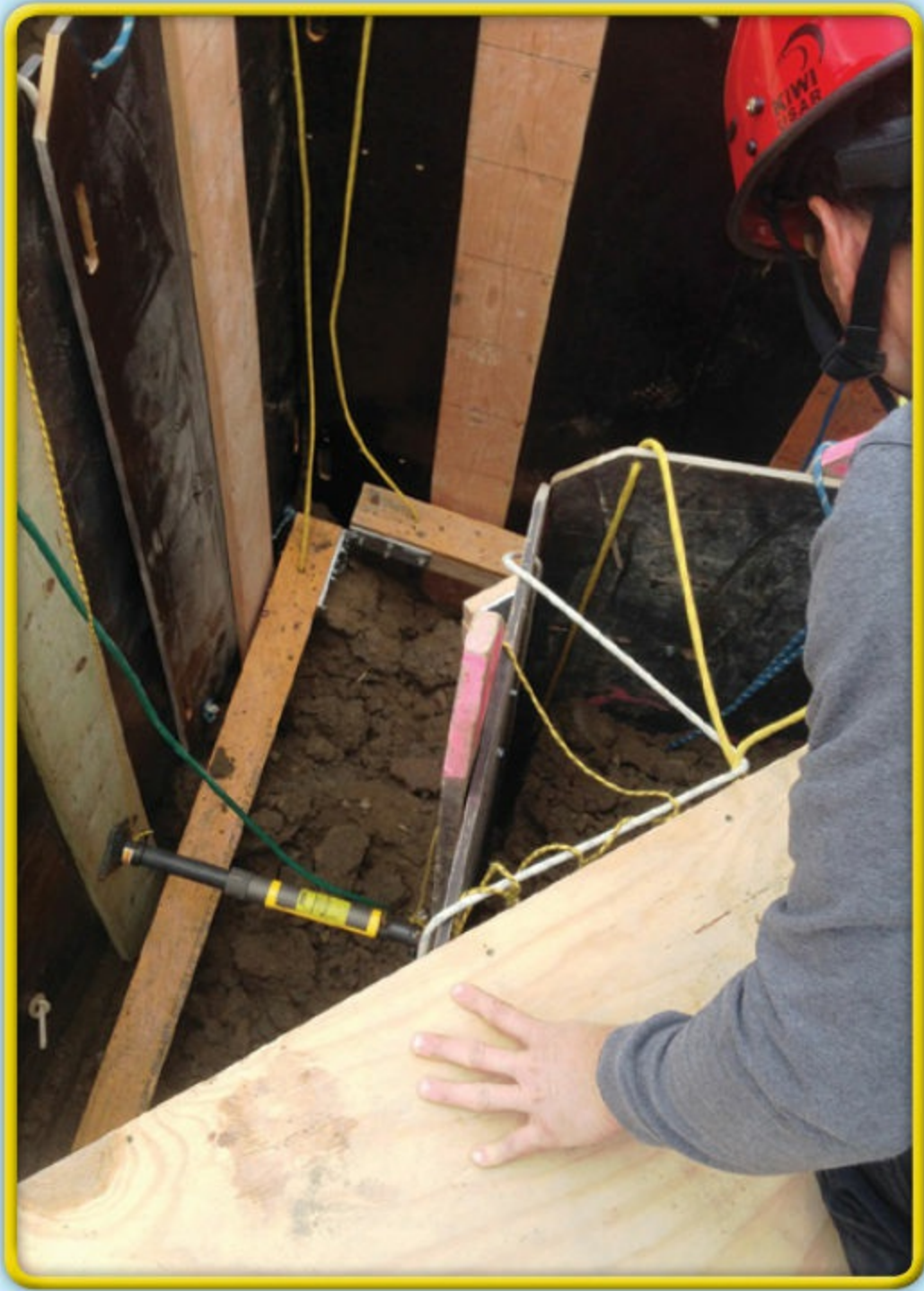
6 Position two panels at the outside corner.
