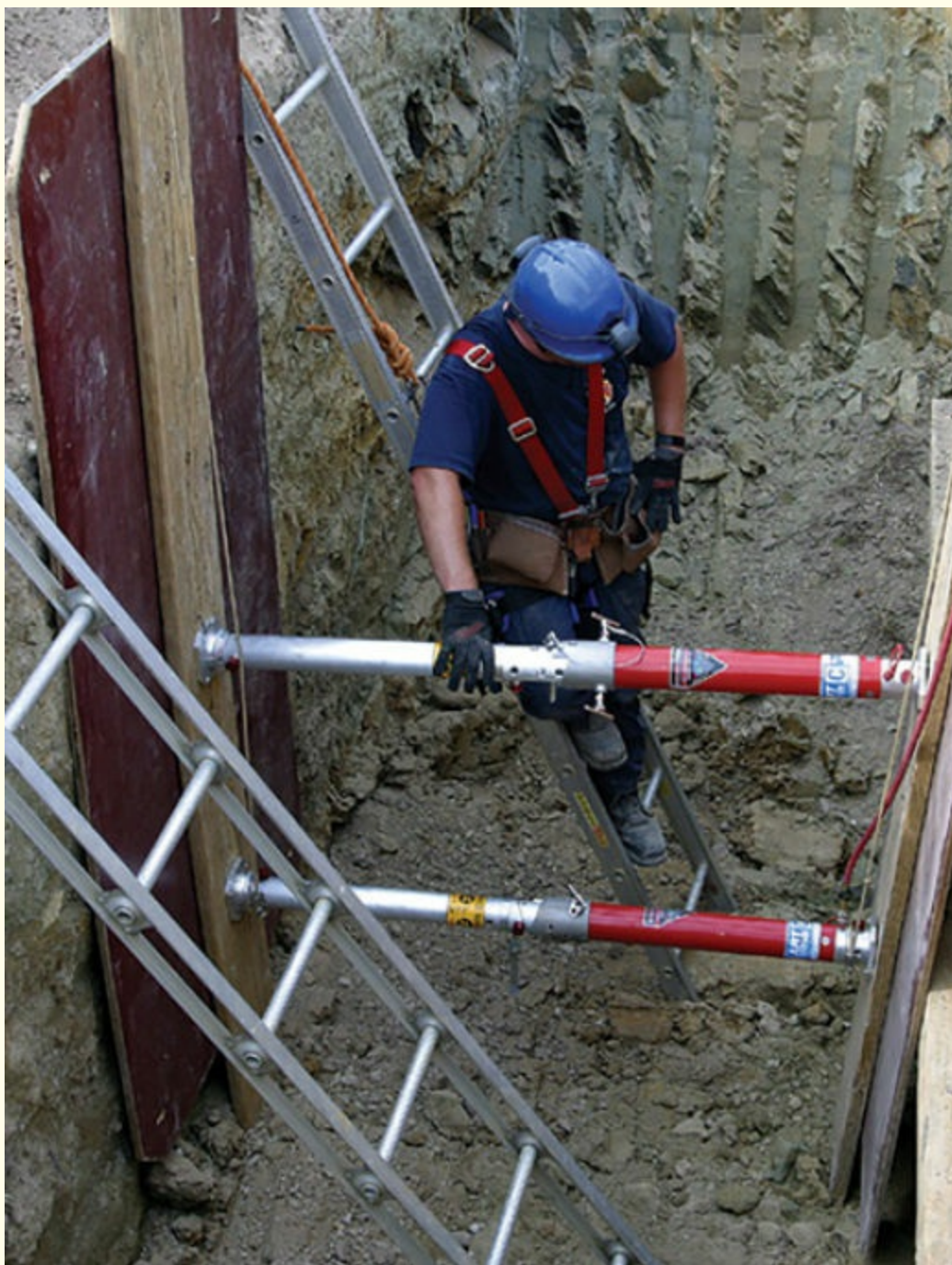
FIGURE 10-7 The bottom shore being installed.
