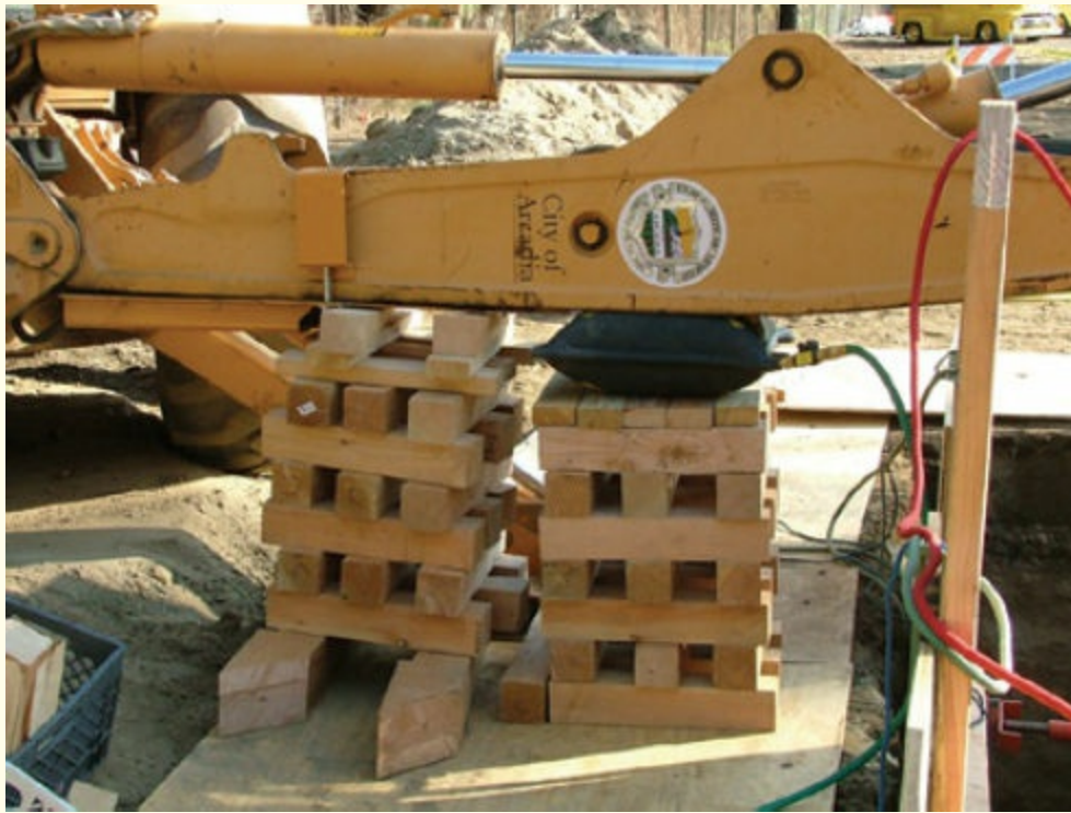
FIGURE 9-16 High-pressure bags lift heavy objects, but only to limited heights.
