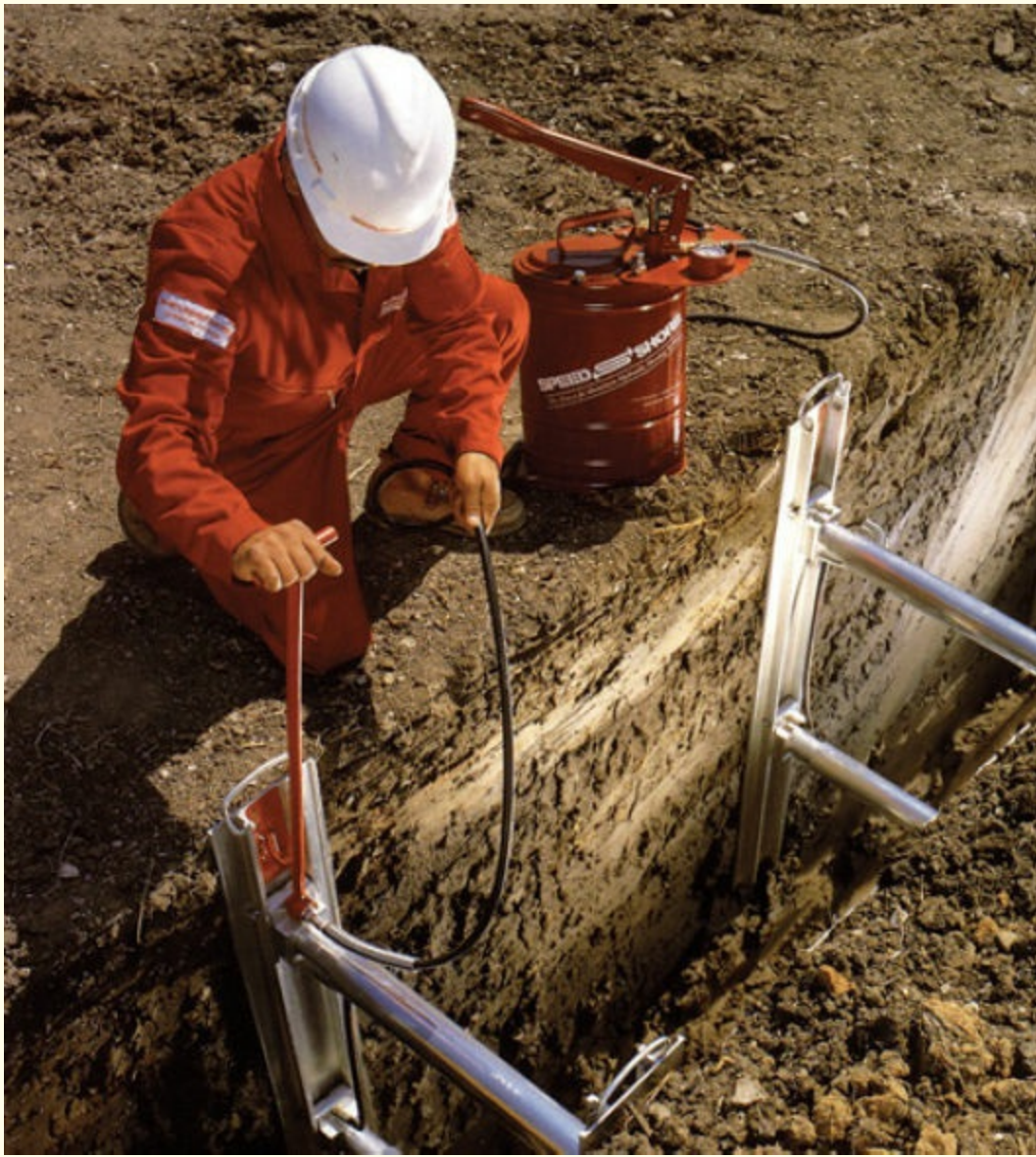
FIGURE 10-3 The Speed Shore has the strongback portion of the protective system already installed as part of the shore. This type of skip shoring is not recommended when soil has collapsed or is active. Courtesy of Speed Shore Corporation
