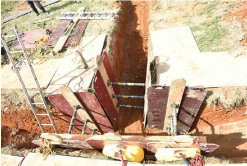
FIGURE 11-13 Complete T-trench rescue shoring.
