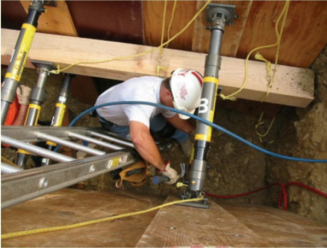
FIGURE 2-1 The rescue personnel who perform trench rescue are specially trained technicians.
