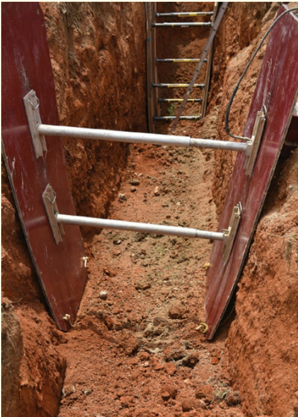
FIGURE 6-15 Hydraulic shores are very popular but are limited in use to walls that are mostly vertical.
