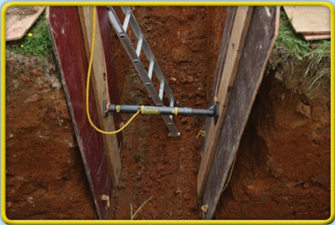
2 Lower a wale to the trench floor on the long wall.
