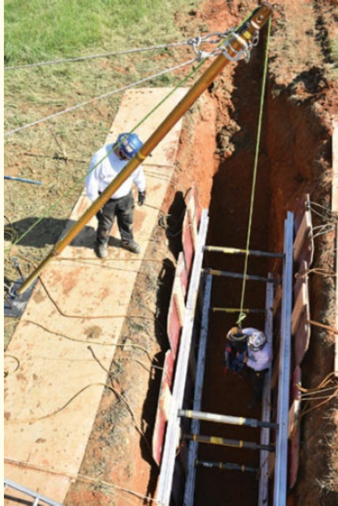
FIGURE 10-12 Inside wales are used to span a trench panel.
