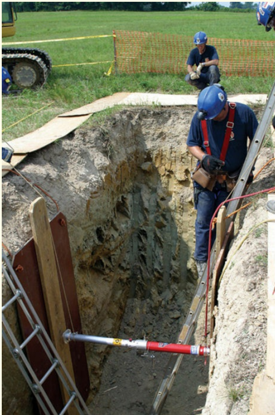
FIGURE 10-6 Middle shore installed on the first set of panels.
