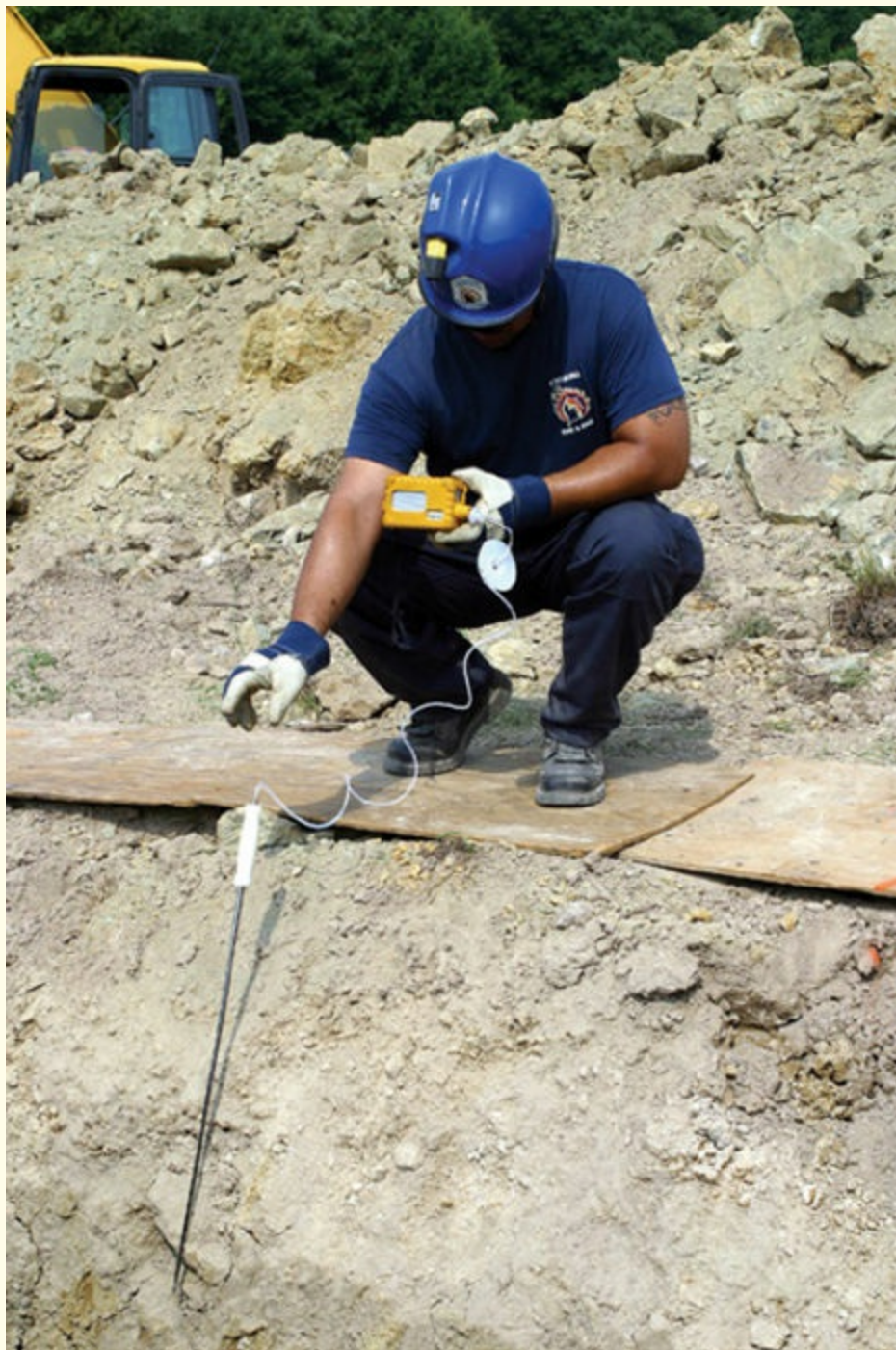
FIGURE 8-8 Atmospheric monitoring should take place on all trench and excavation rescues.
