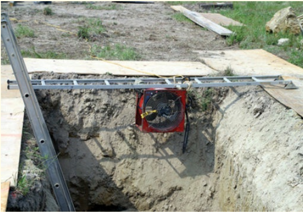
FIGURE 6-22 Placing a piece of tape on a ventilation fan can provide a visual indication of when it is working. © Jones and Bartlett Publishers. Courtesy of MIEMSS.
