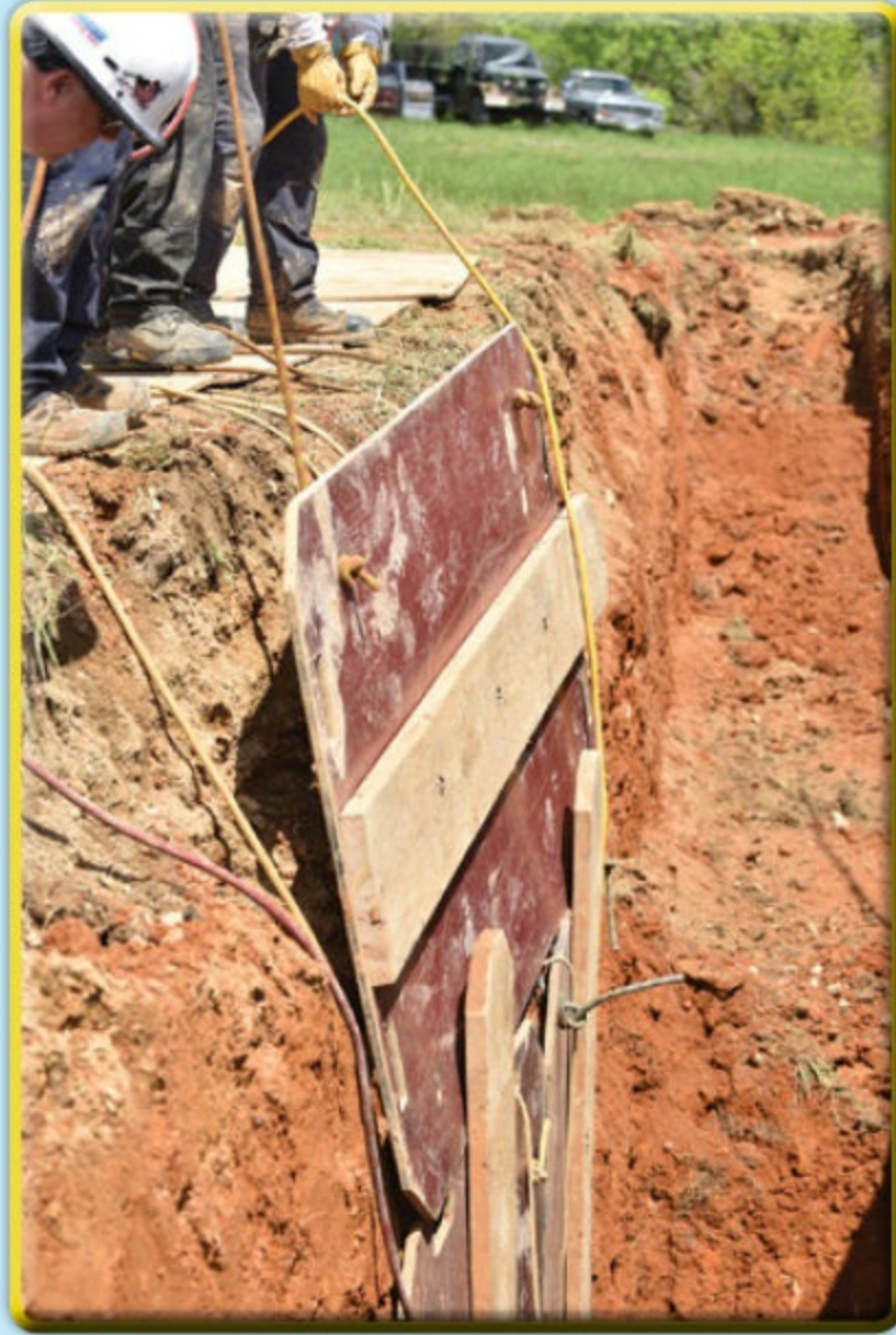
6 Position the top panels (horizontal for a 12-foot [3.7-m] deep trench).
