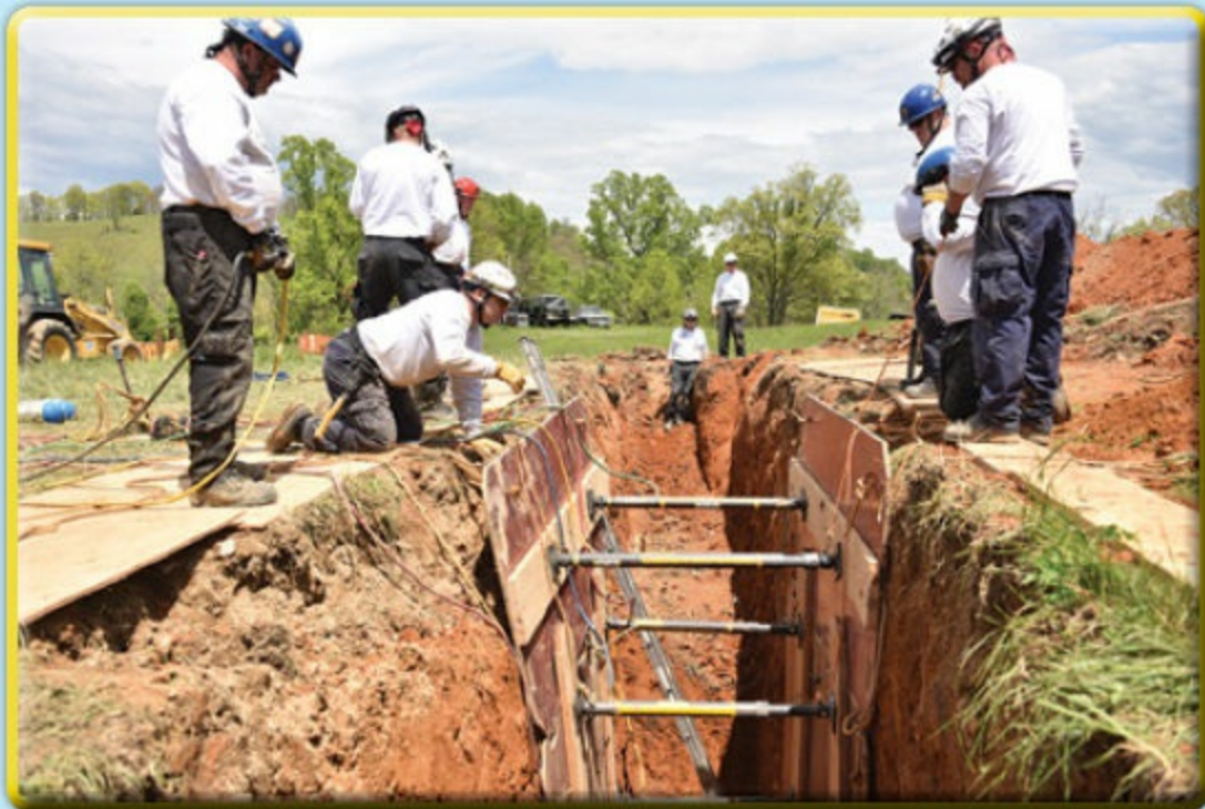
6 Position the top panels (horizontal for a 12-foot [3.7-m] deep trench).
