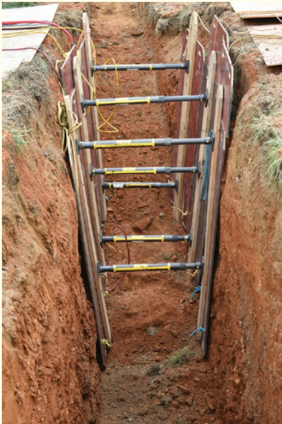
FIGURE 11-3 The three-panel set in a straight-wall trench.
