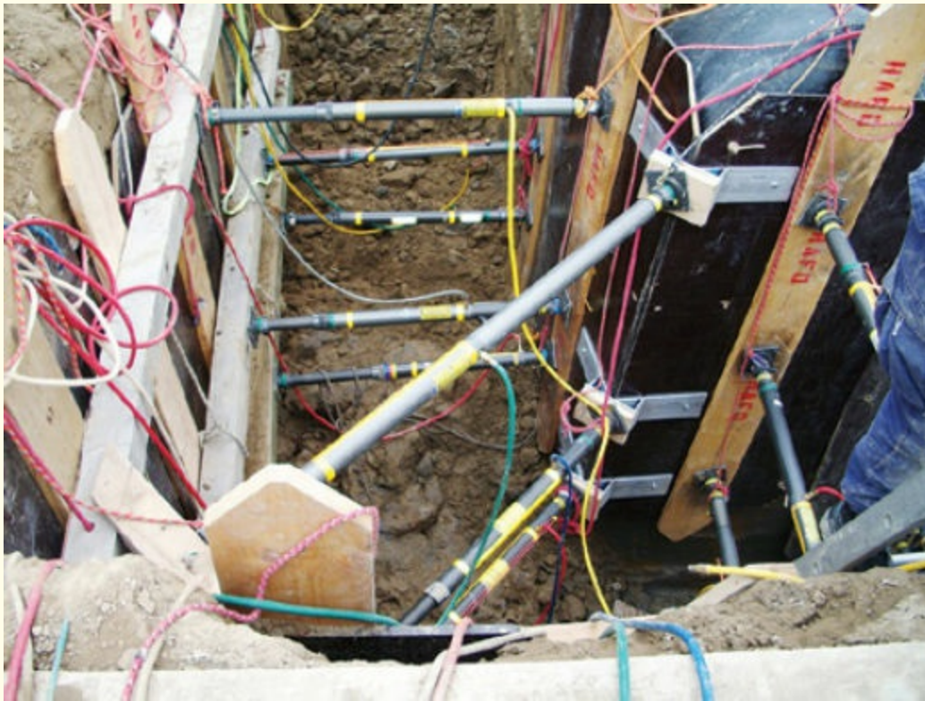
FIGURE 11-17 Deeper L-trenches require additional tiers of struts. Courtesy of Ron Zawlocki
