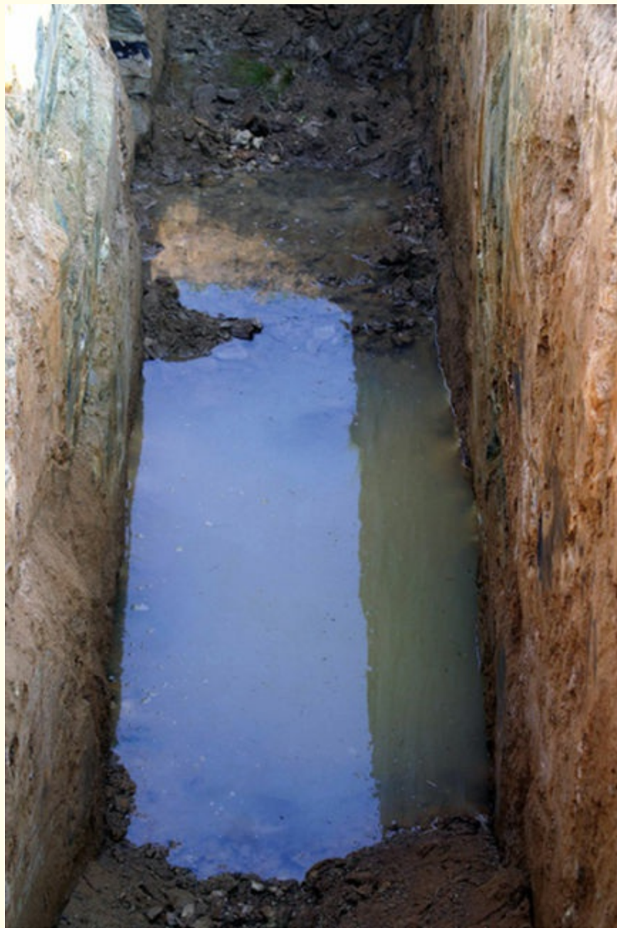
FIGURE 4-8 Minimize the effects of water in the trench by dewatering; however, be mindful that water-saturated soil may continue to present hazards to rescue personnel and increase the soil's lateral forces.
