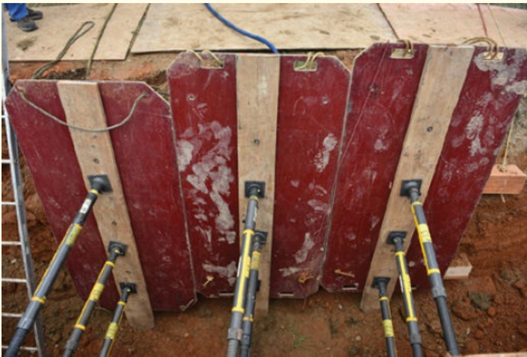
FIGURE 11-5 Completed outside wale trench shoring.
