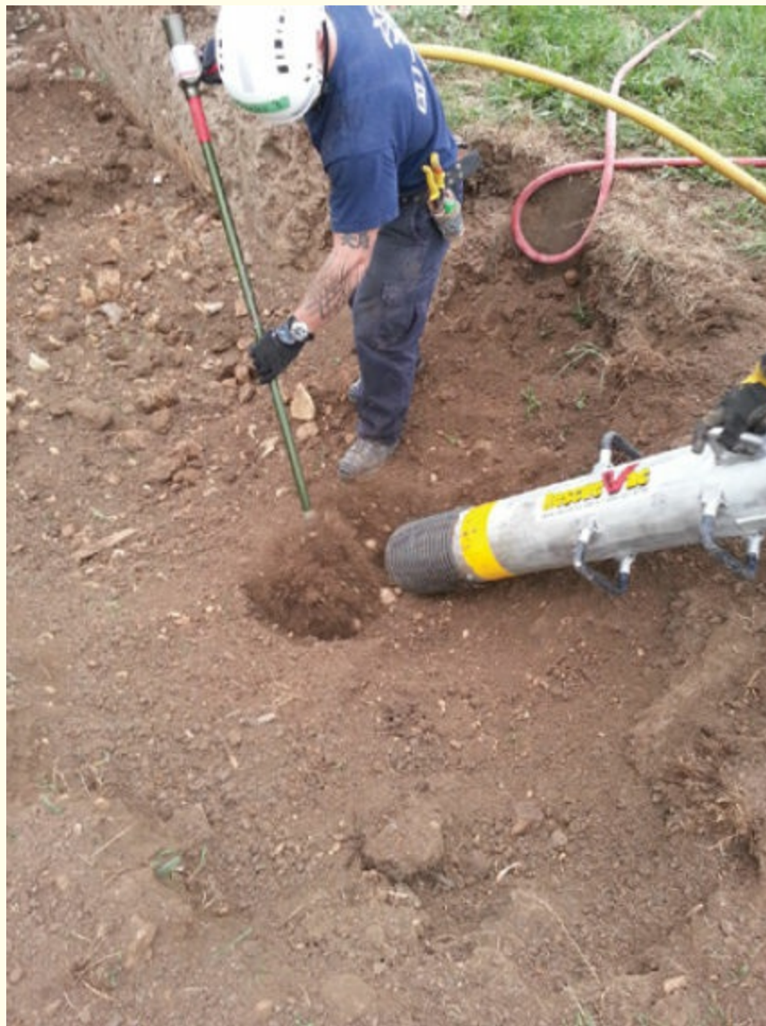
FIGURE 12-13 The air knife uses compressed air to reduce the size and change the consistency of soil so that it can be vacuumed more easily. Courtesy of Rescue Vac
