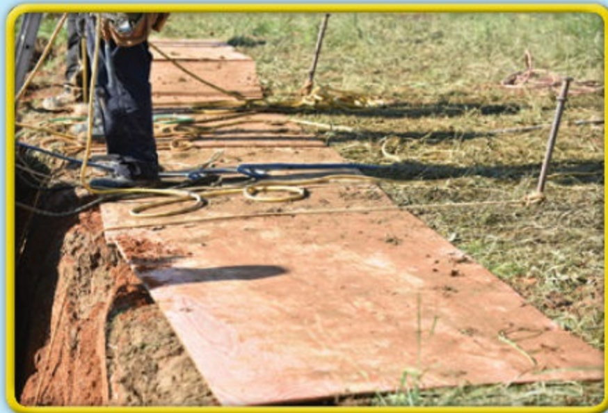
7 Install two pickets behind the lip on the long wall side.
