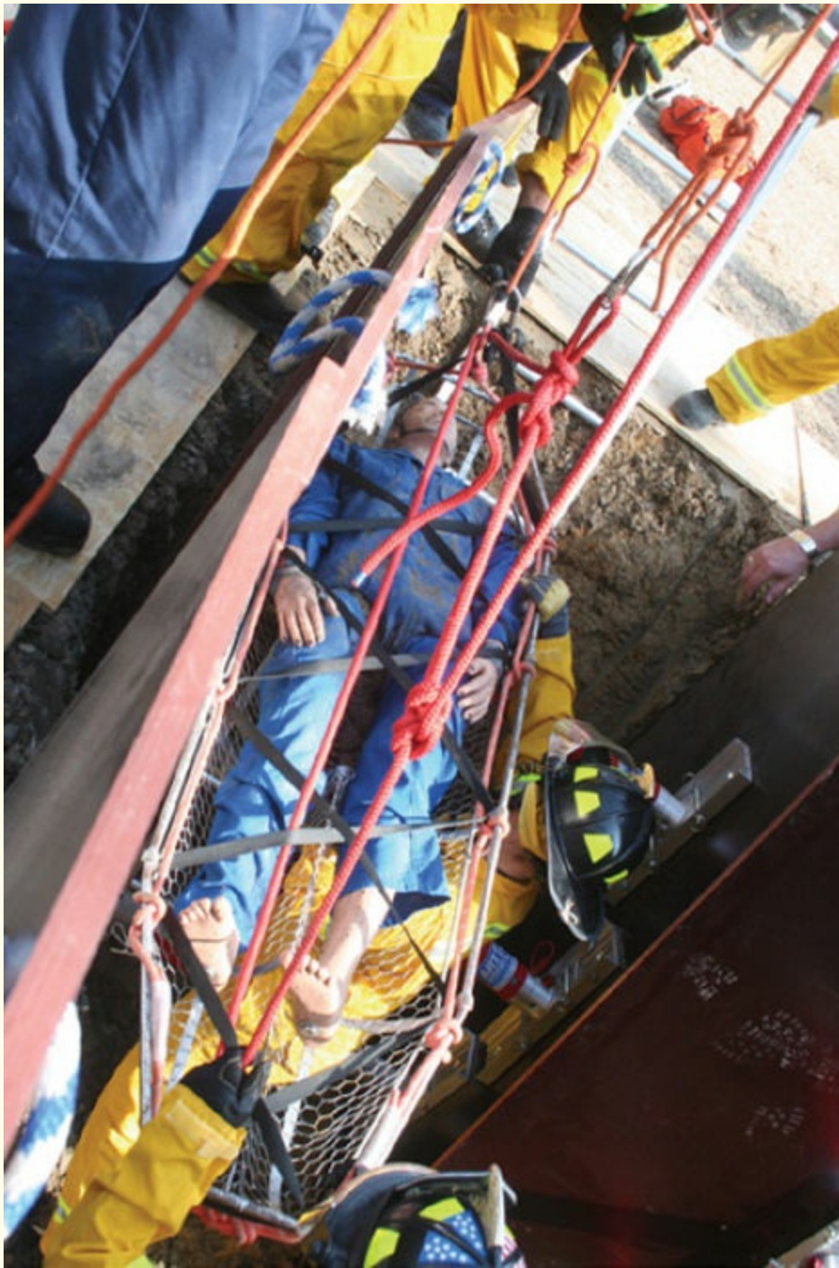
FIGURE 12-18 The vertical lift is usually the preferred method for removing victims from a trench. Courtesy of Lance Cpl. Angel J. Velasquez/U.S. Marines
