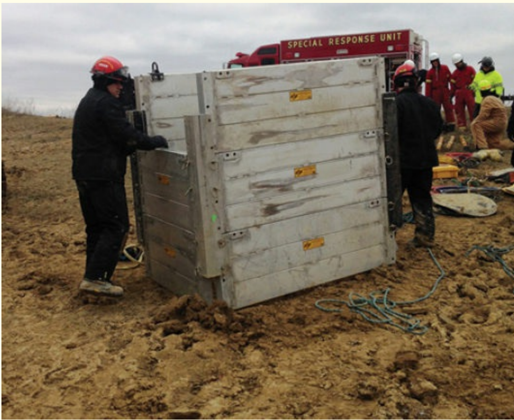
FIGURE 10-14 Modular shield. Courtesy of Ron Zawlocki
