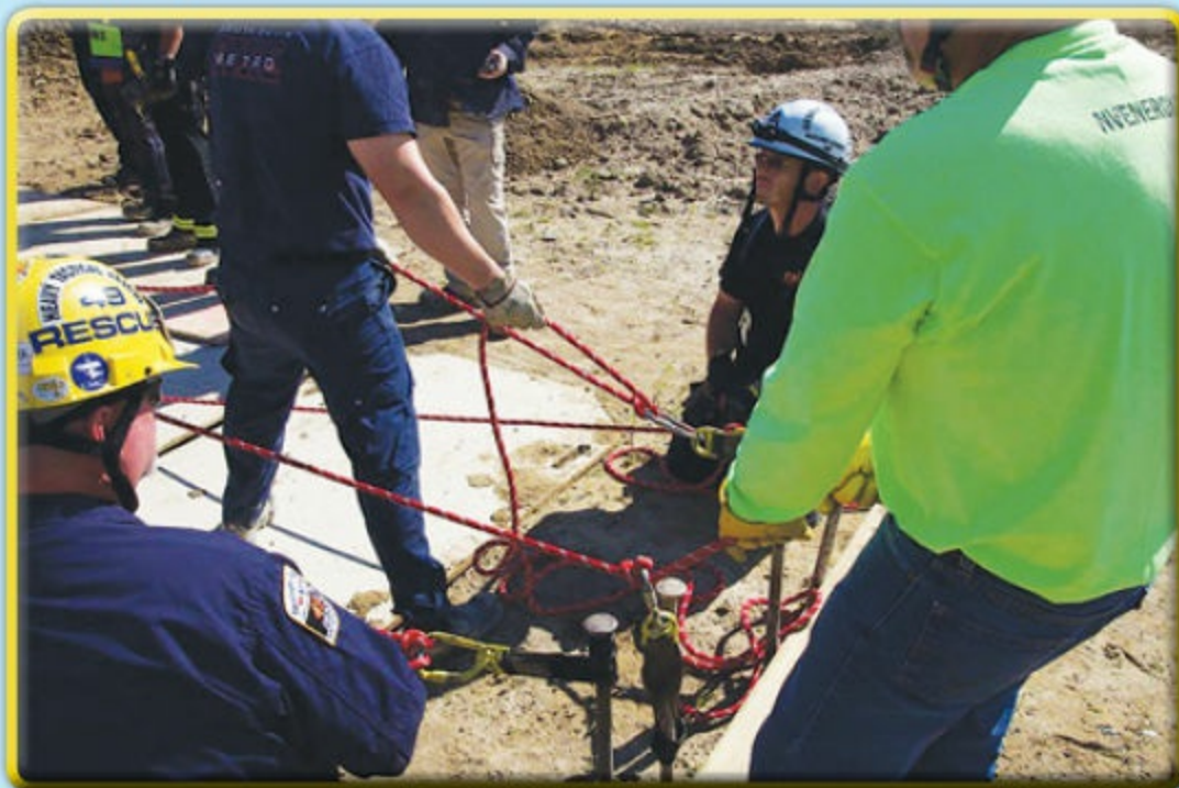
3 Nail 2 × 6-inch bracing to the rakers. Courtesy of Ron Zawlocki
