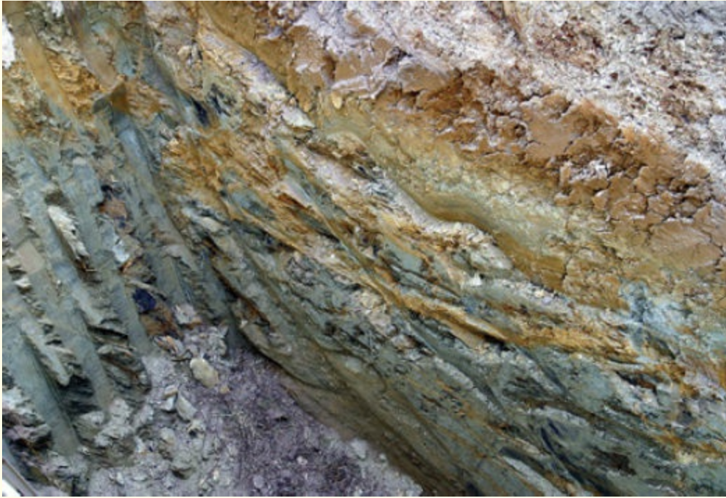
FIGURE 4-7 Layers of varying types of soil should be identified as having an increased collapse potential.
