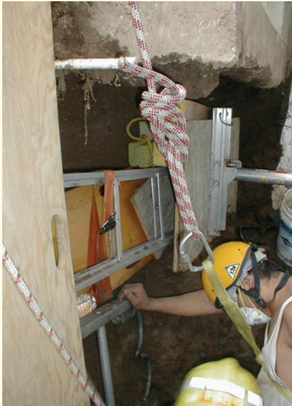
FIGURE 6-23 Although not the preferred method, ladders can be used as wales when 6 × 6-inch or 8 × 8-inch material is not available or access is difficult.
