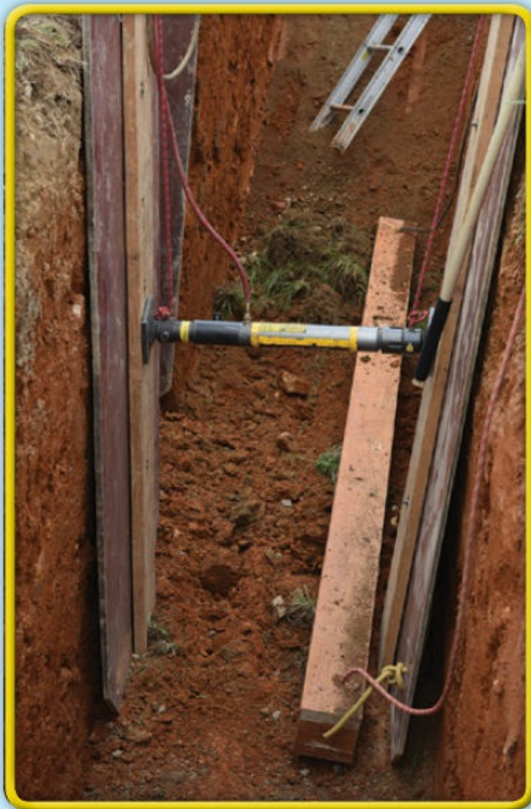
2 Lower a wale to the trench floor on the long wall.
