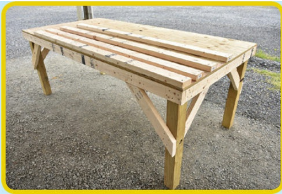
14 The cutting station table is now complete.
