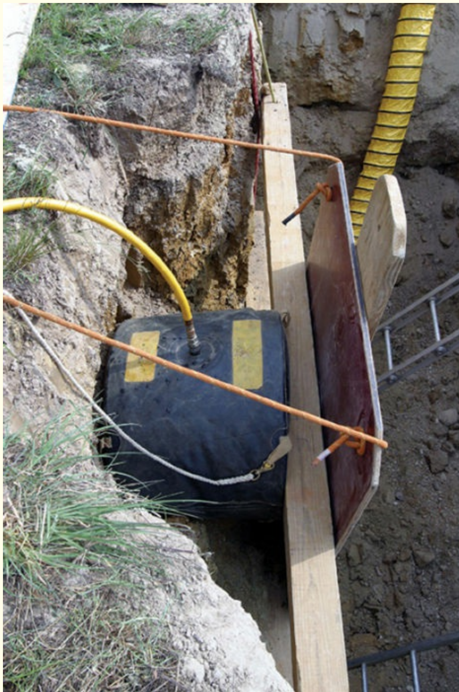
FIGURE 9-19 Low-pressure air bag being used to fill a slough void.
