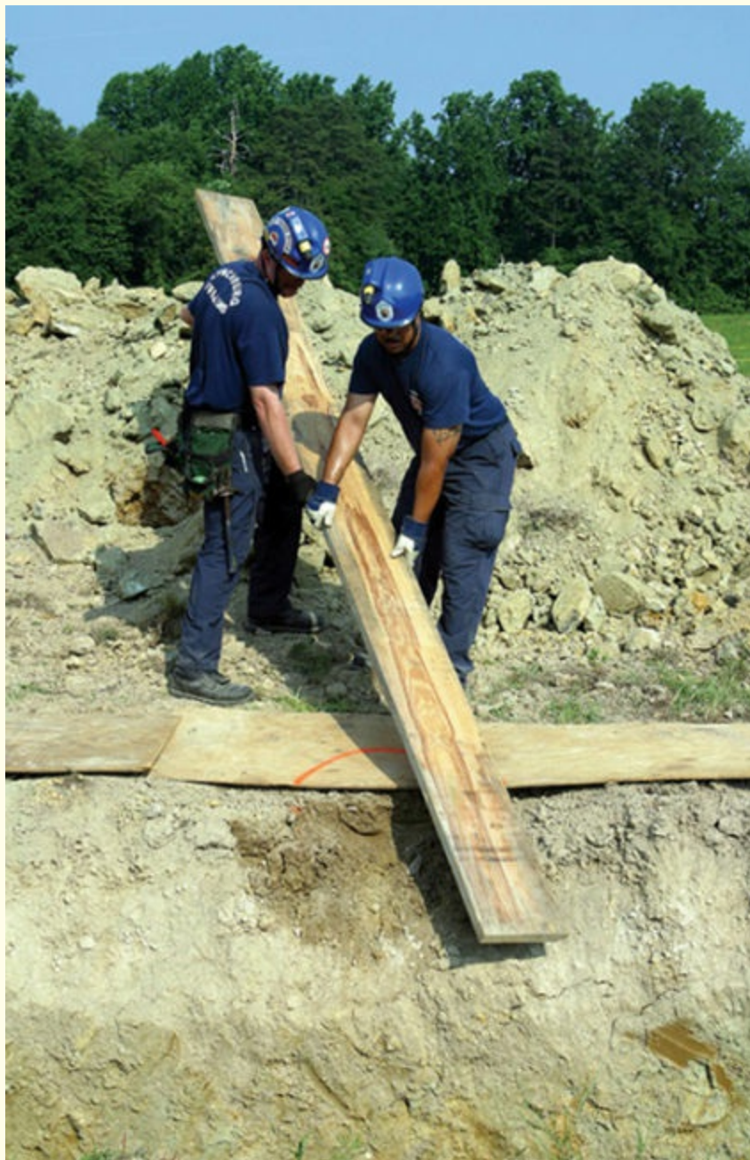
FIGURE 10-5 In hard-packed soils, the strongback can be used without the panel. This type of skip shoring is not recommended when soil has collapsed or is active.
