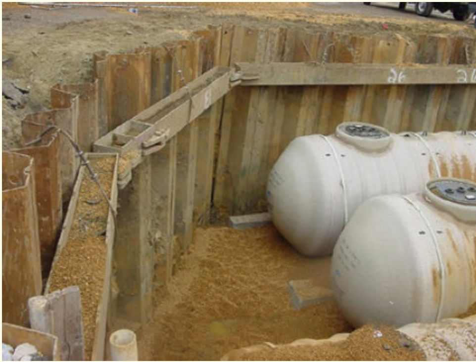
FIGURE 10-20 Interlocking steel sheet pile shoring is a commercial technique typically used in deep trenches subject to tremendous compressive forces. These are seldom used at rescue incidents.
