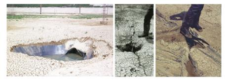
Fig. 19 Reservoir bottom (Hutovo, Herzegovina). Collapse and cracks beneath the geomembrane
