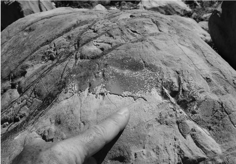
Figure 13. Corrosion of a limestone slab. A trail blaze in waterproof paint has protected the underlying limestone from dissolution of about 1 mm over 30 years. Photo taken on a trail midway up a mountain in a Mediterranean climate.
