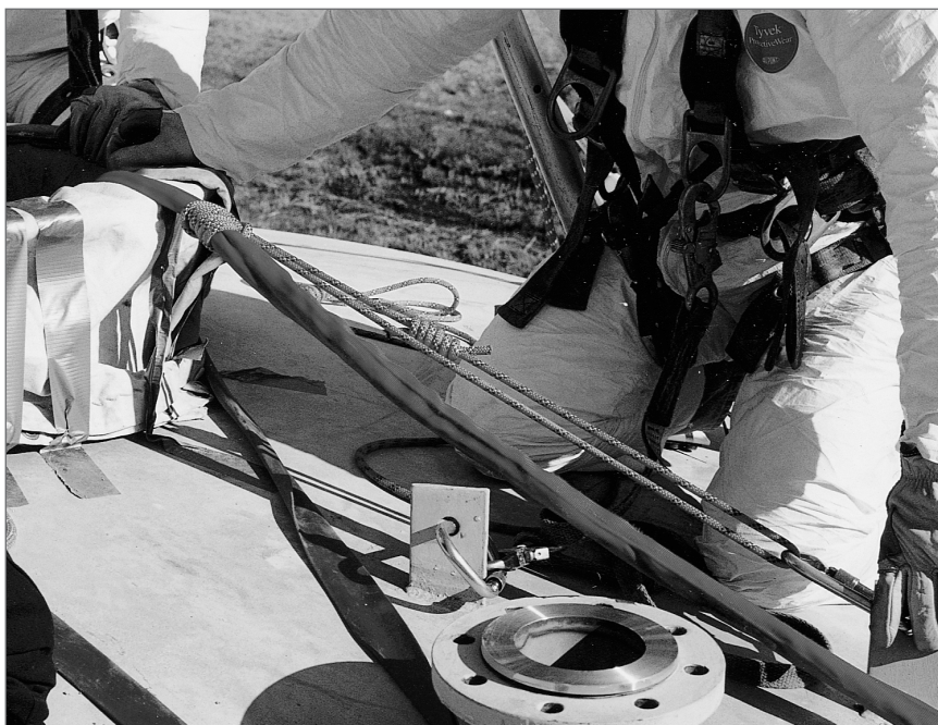
Using a slip knot to manage the deployment of a sheathed umbilical.
