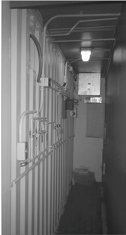
A lockout, tag-out wall at the FDNY training facility.
