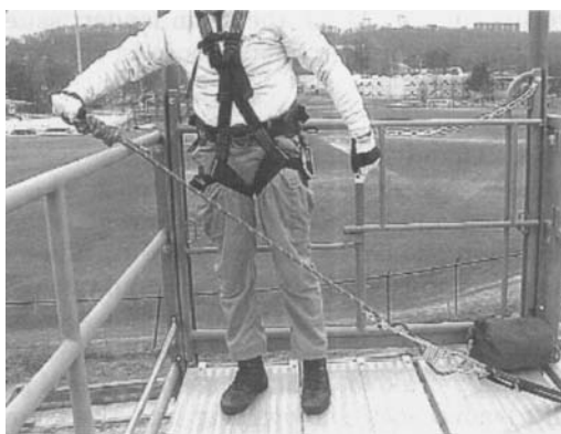
Figure 17.13 In preparation for a low-point lower, index the lowering line in relation to the edge before the descent control device is roped in or the lowering line is attached to the load.
