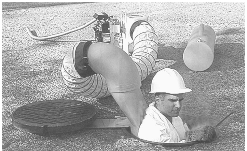
Figure 6.19 The Saddle Vent ® by Air Systems International is one example of equipment used to conduct ventilation air into a space without obstructing the entry/exit point. (Photograph courtesy of Air Systems International.)
