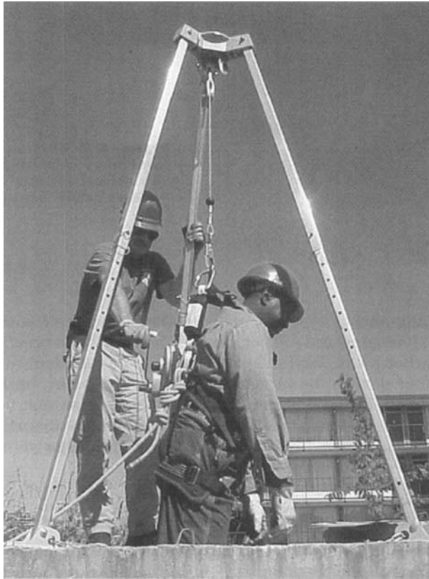
Figure 13.2 Tripods are temporary portable anchors engineered to hold a specific working load.
