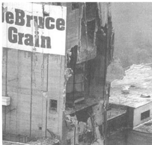
Figure 3.8 The DeBruce grain elevator, and world’s largest, exploded when dust in the underground tunnels was ignited by a spark from an unlubricated conveyor belt roller.
