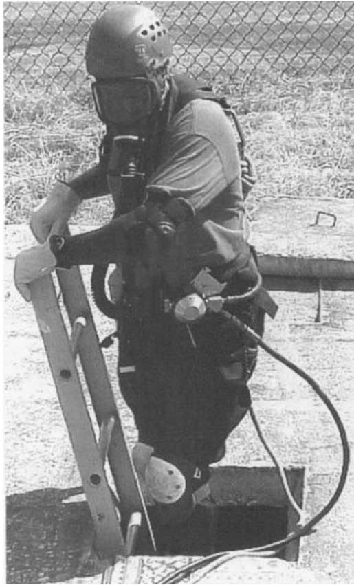
Figure 7.5 Supplied-air (airline) respirators provide breathable air to the entrant from a source outside the space.
