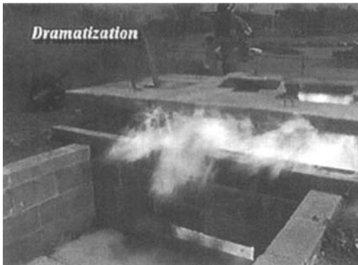
Figure 1.10 A potentially flammable atmosphere within a confined space is a permit-required condition.
