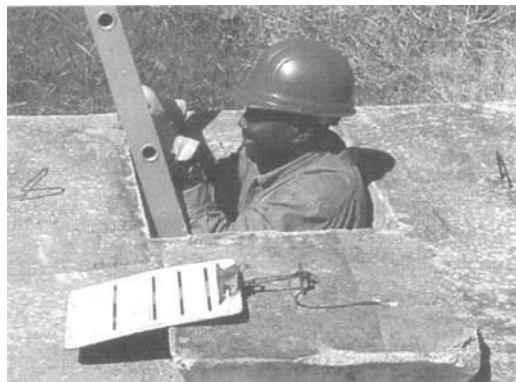
Figure 1.8 Confined space configuration restricts the entry and exit of the entrant.
