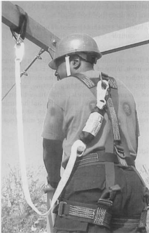
Figure 14.7 A simple fall-protection system can be rigged with a class III harness, fall-arrest lanyard with shock absorber, and an anchor.
