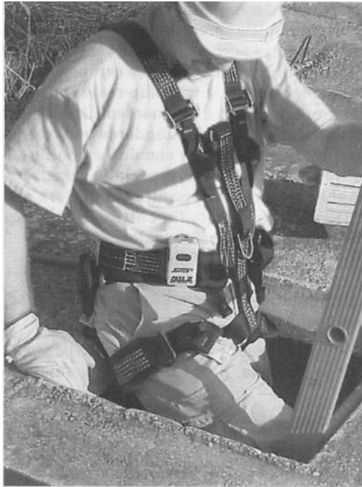
Figure 14.5 The personal alert safety system (PASS) device activates automatically if the wearer remains immobile for a specific length of time, and makes lost or incapacitated entrants much easier to locate.
