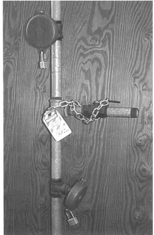
Figure 6.24 A double block and bleed is performed by locking two in-line valves in the closed position and locking a vent valve located between the two closed valves in the open position.
