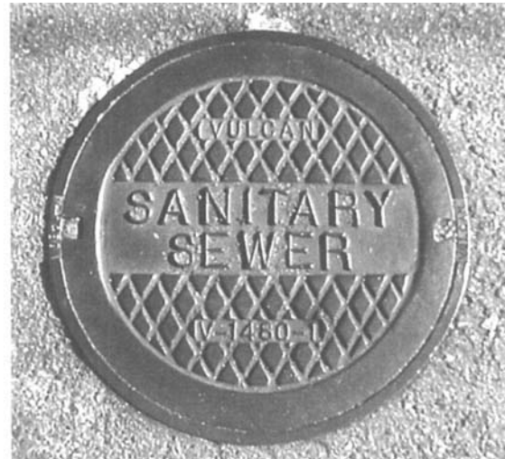
Figure 1.4 Sewers, including sanitary and storm sewer systems, are very common confined spaces in urban and suburban areas.
