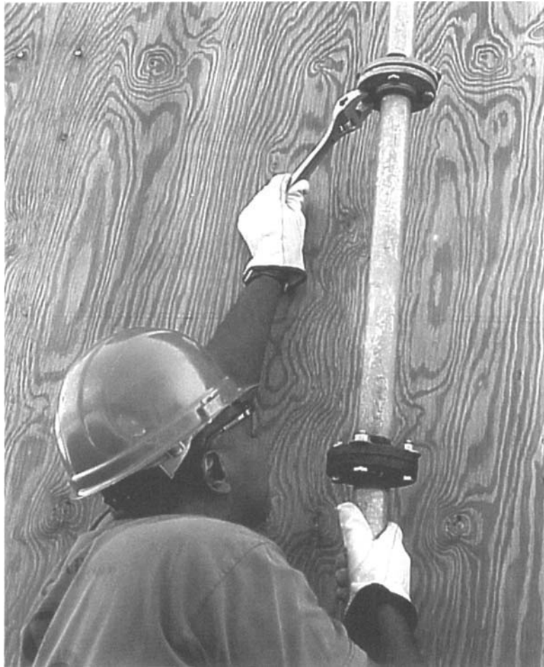
Figure 9.1 Head protective helmets protect the head from impact and penetration by falling objects.
