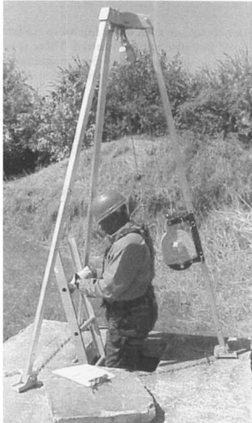
Figure 14.11 The winch on this tripod has a fall-arrest setting that allows cable to feed out smoothly under normal conditions but locks if a fall occurs.
