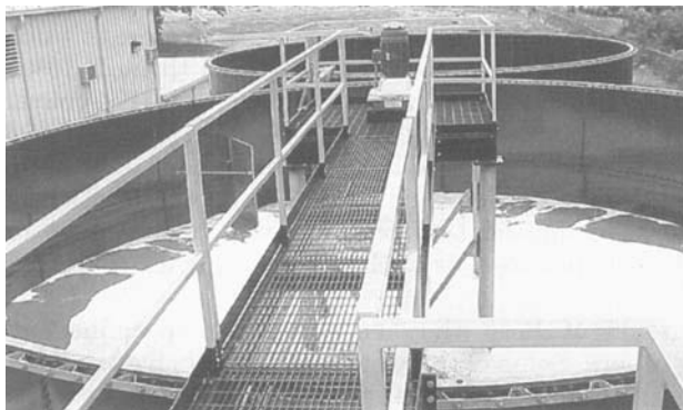
Figure 1.5 Open-top structures such as vats, pits, and diked areas around storage tanks may be classified as confined spaces.
