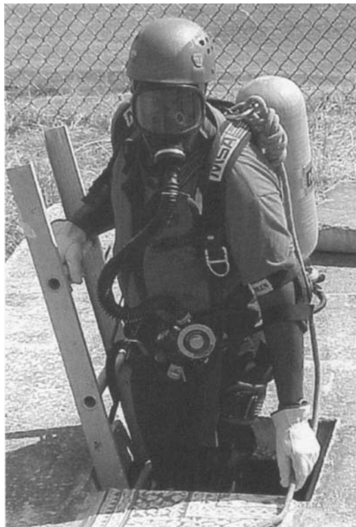
Figure 7.6 The self-contained breathing apparatus provides the highest level of respiratory protection and allows the entrant to move around without airline restrictions.
