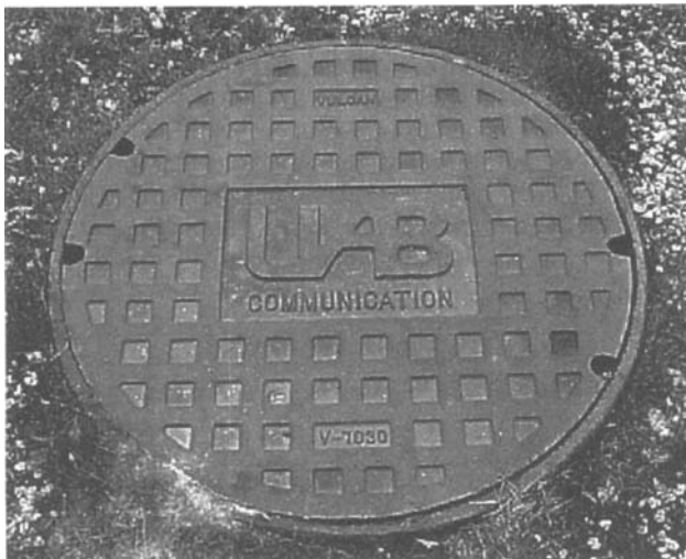
Figure 1.3 Vaults are common confined spaces in industries involving telecommunications, oil and gas transmission, and electrical transmission.
