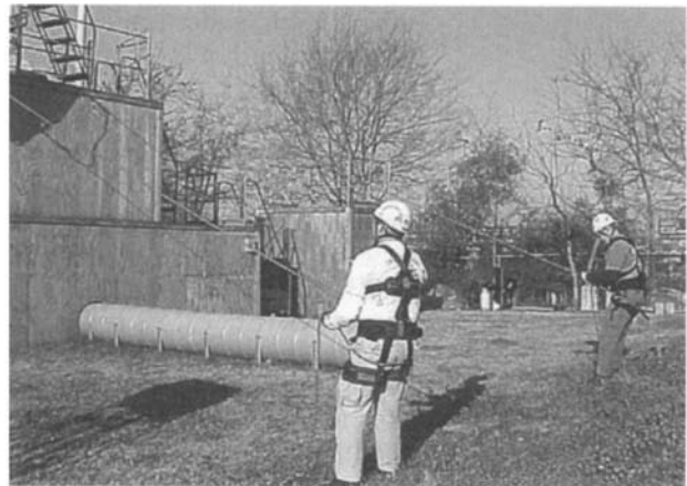
Figure 18.34 Tag-line tenders guide the litter to keep it clear of the side of the structure during lowers.
