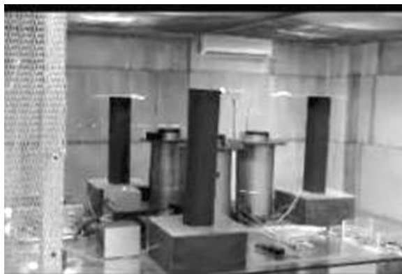
Fig.70. 100 kW three phase generator in Turkey.
